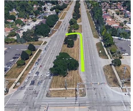
An RCUT intersection has no left turns. A "J-turn" lane (yellow) provides access to the opposing lane and a safer right turn.
