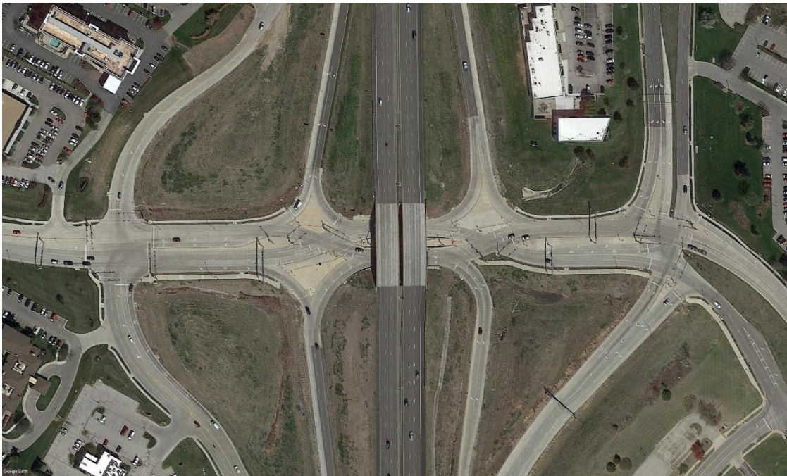
Figure 9-6: Example of a DDI with a relatively short crossovers' distance (I-29 & Tiffany Springs Pkwy, Kansas City, Missouri)
