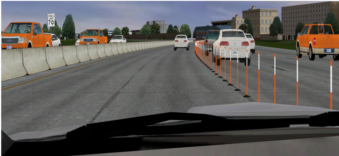
Figure 3-6: Orange Delineators with White Reflective Sheet and Concrete Surface
