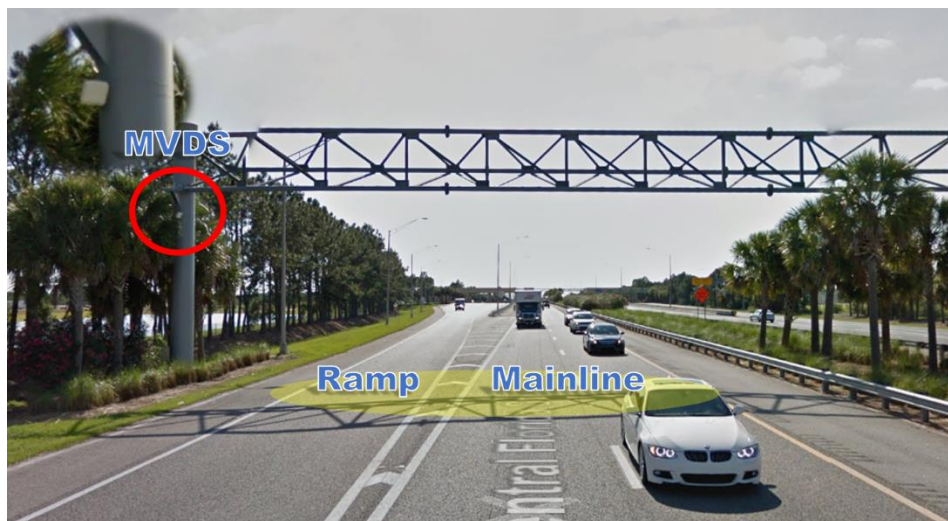
Figure 62. Example of MVDS installation and lane type distinction
