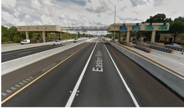
(a) Mainline toll plaza
