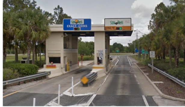
(b) Toll gate on on/off ramp
