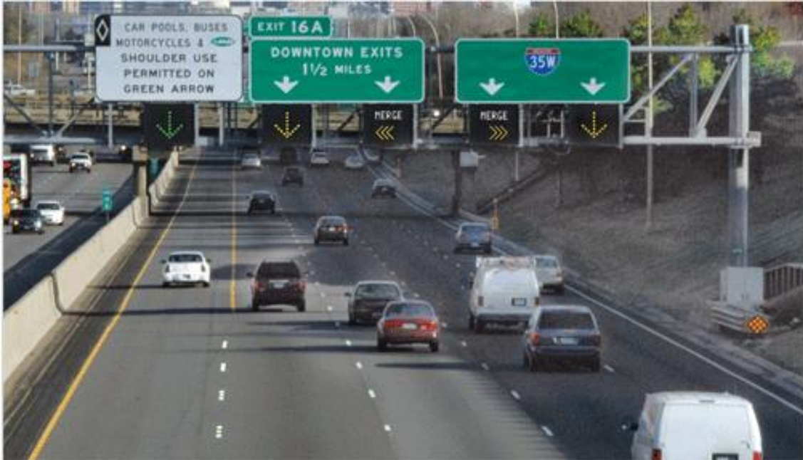
Figure 5. Intelligent lane control signals on I-35W
