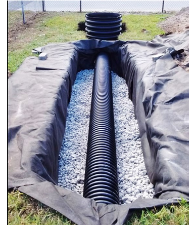
Geotextile wraps around a French drain.
