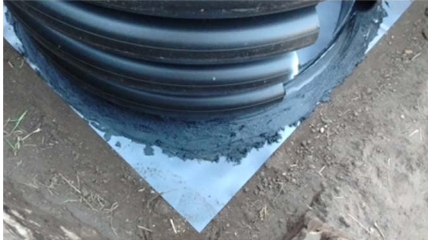
Figure 3.42: Sealing the sump
