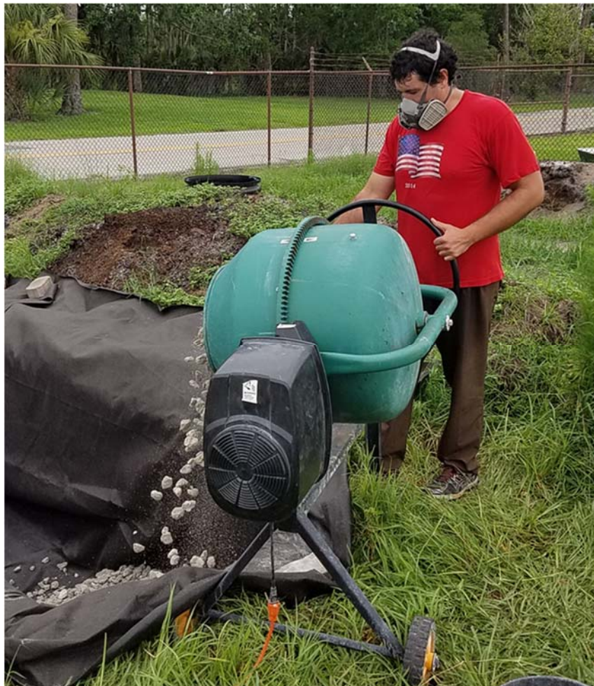
Figure 3.43: Mixing fines and aggregate
