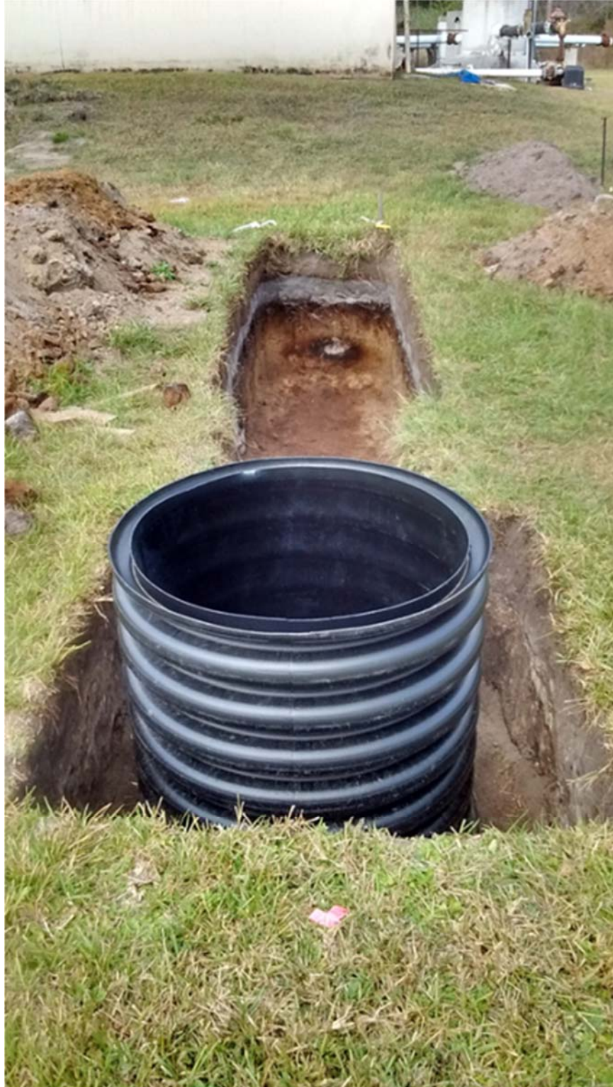
Figure 3.41: The sump placed in the trench
