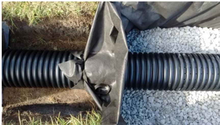
Figure A2. End cap (up) and start of French drain (bottom)
