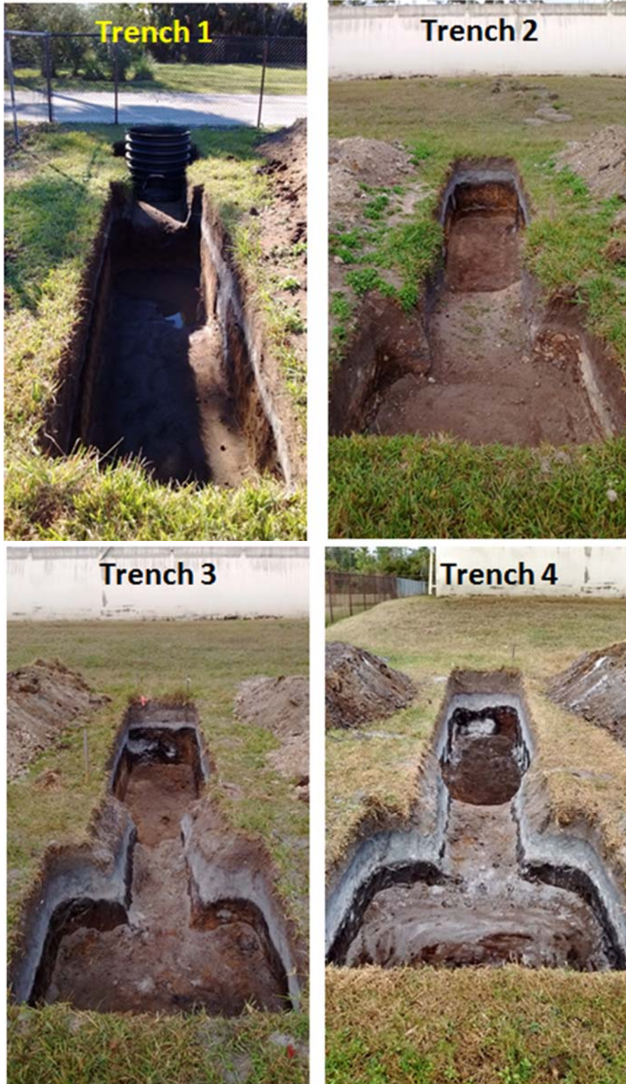
Figure A1. Photos of four trenches
