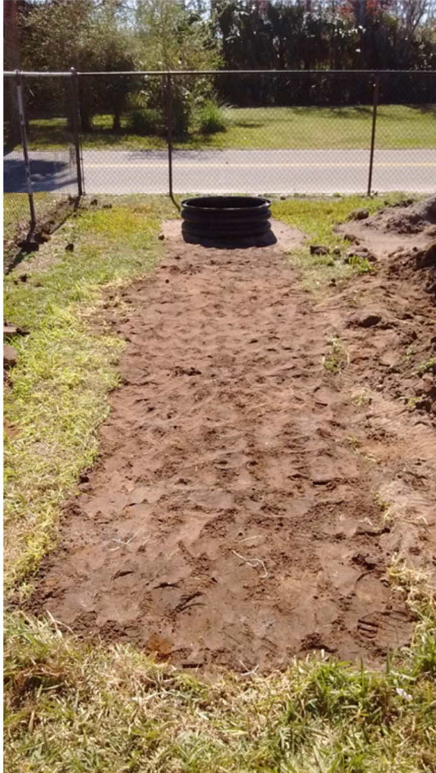
Figure 3.47: Completion of French drain 1 (RCA "as is") construction
