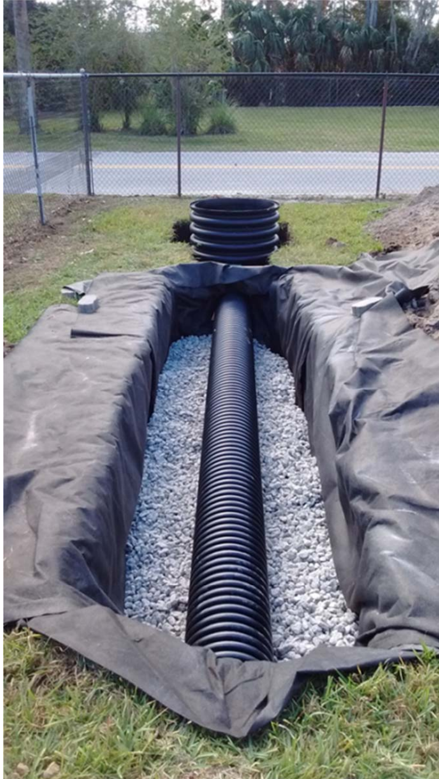
Figure 3.45: Placement of HDPE pipe in trench
