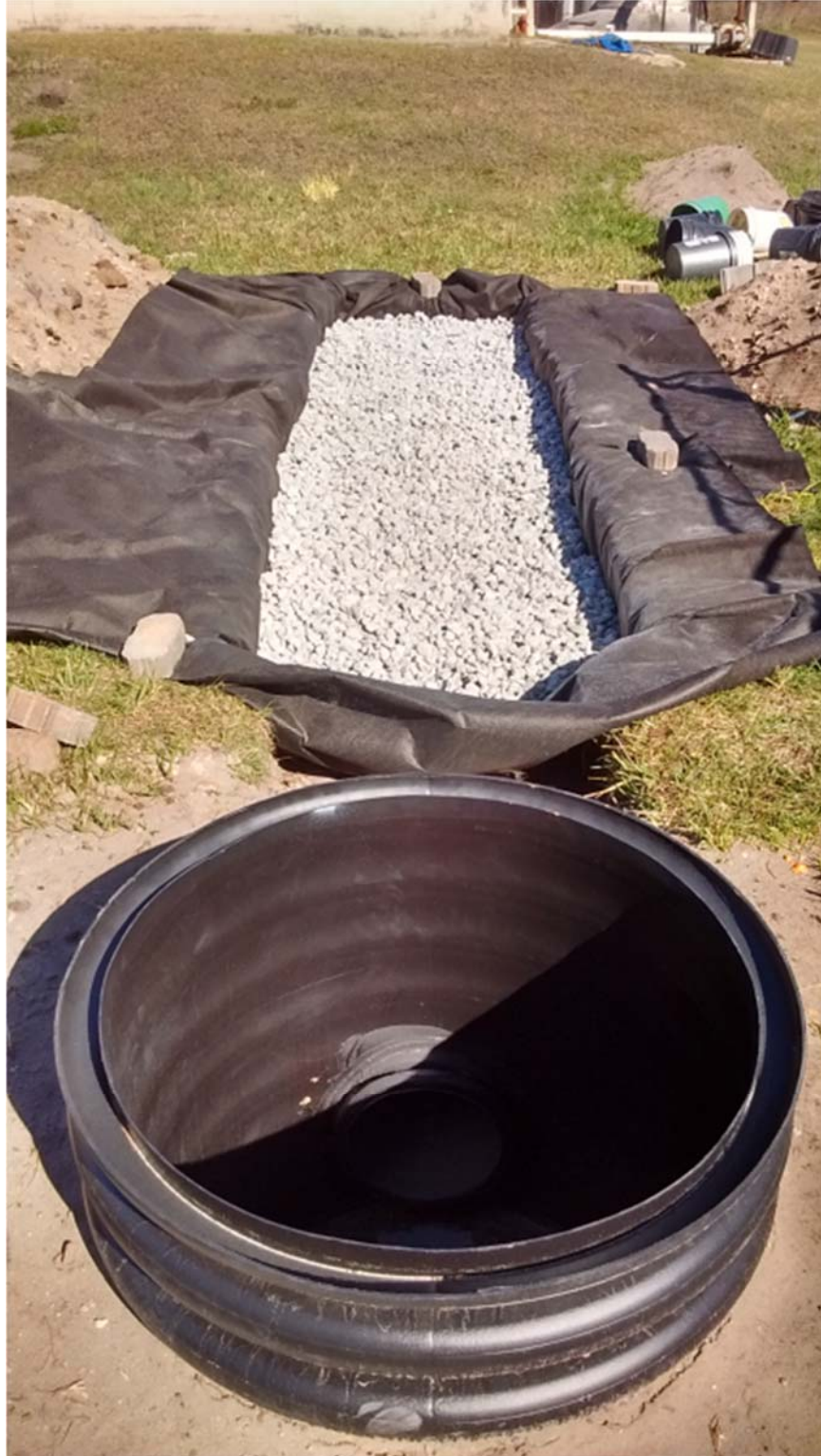
Figure A4. Construction of French drain
