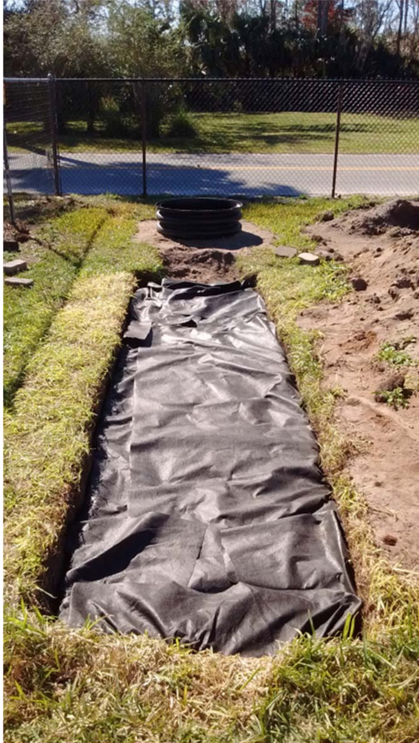
Figure 3.46: Geotextile covering aggregate
