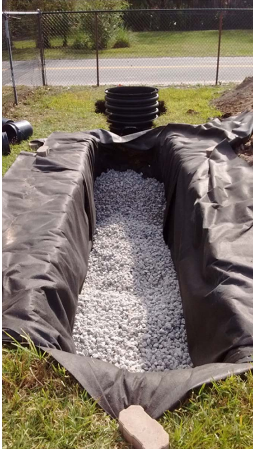
Figure 3.44: Placement of aggregate in trench
