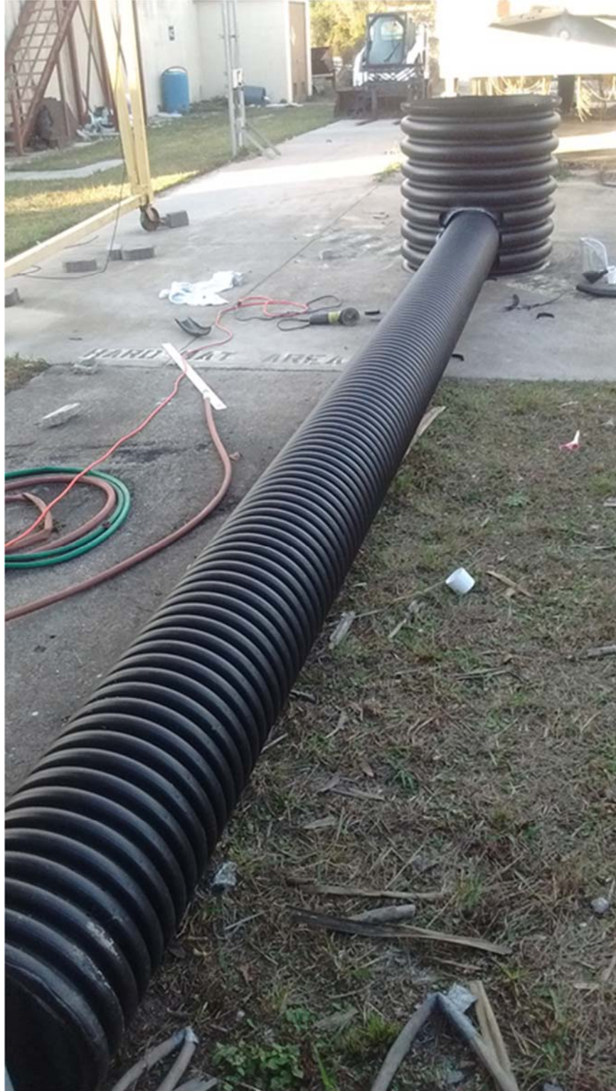
Figure 3.40: French drain plumbing
