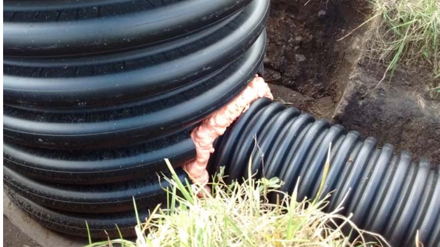
Figure 3.34: Sump-French drain interface
