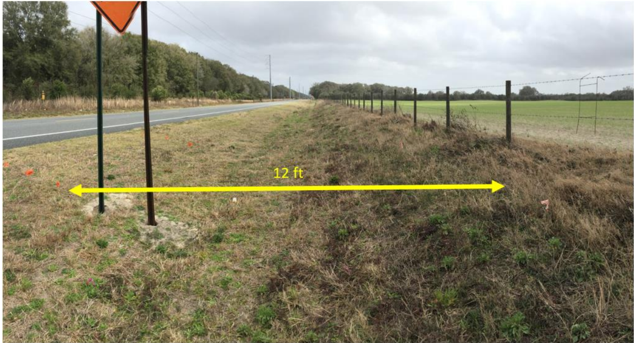
Figure 35. Linear ditch construction site
