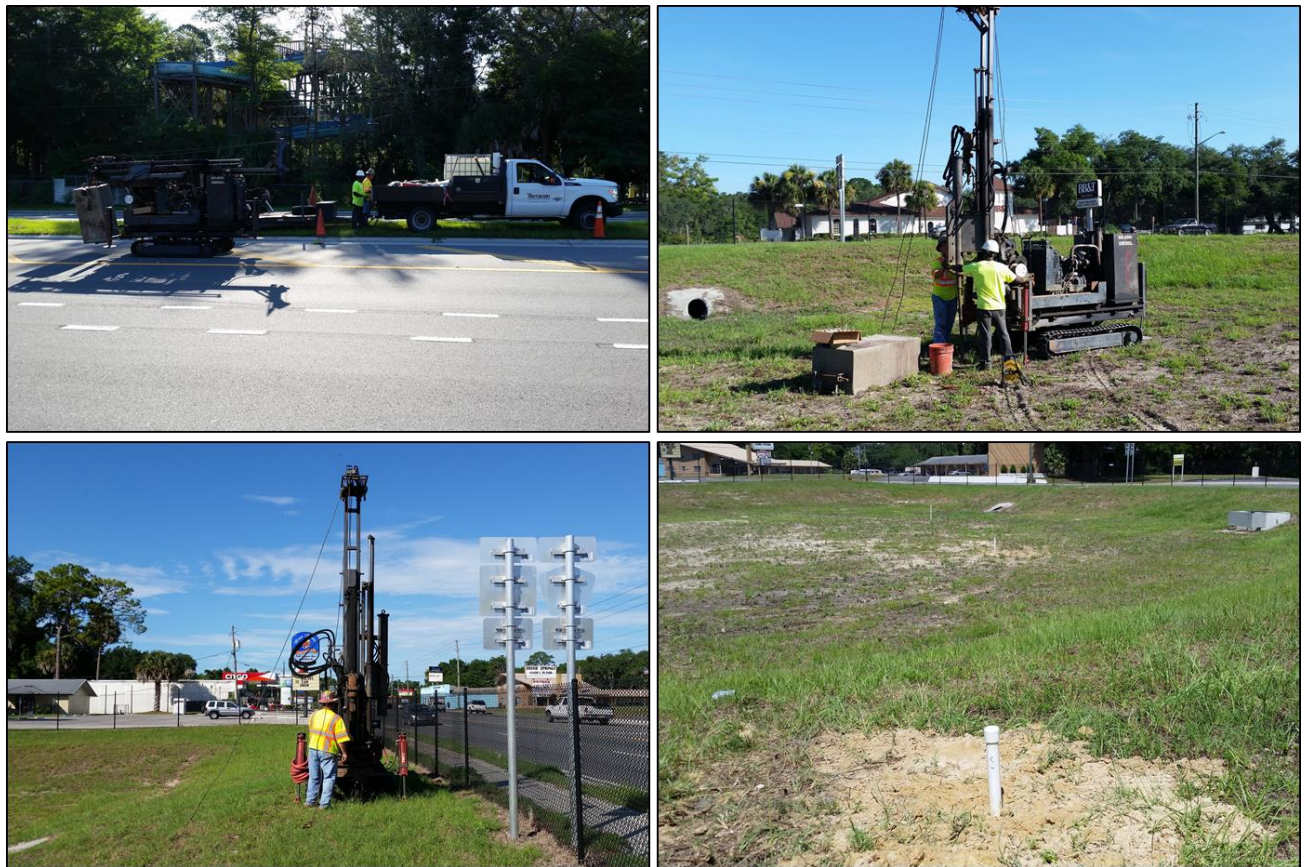
Figure 14: SPT and well installation at SR 35 Basin 9b
