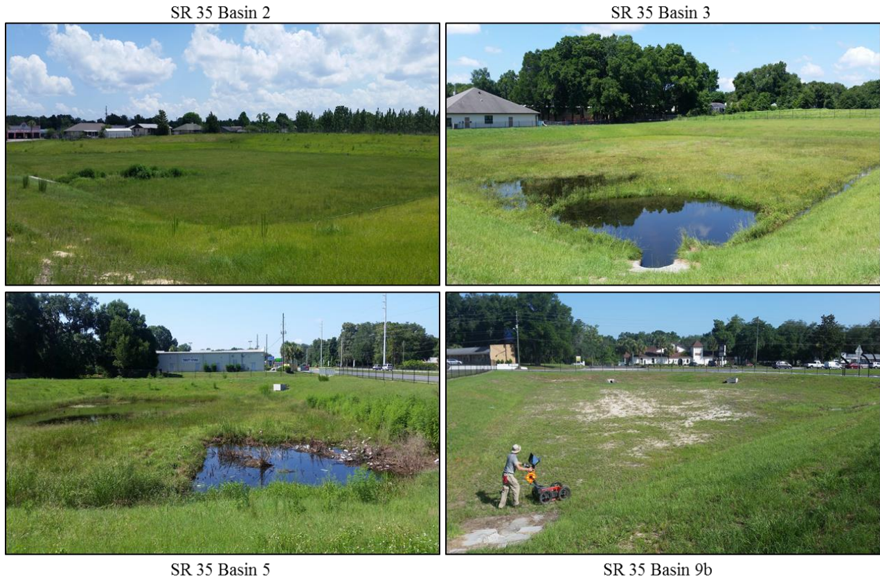
Figure 9: Basin conditions during GPR investigation
