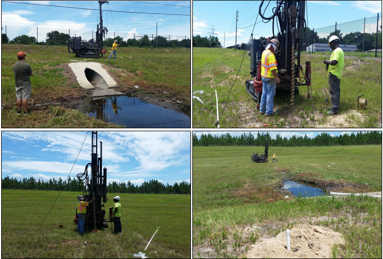
Figure 15: SPT and well installation at SR 35 Basin 2
