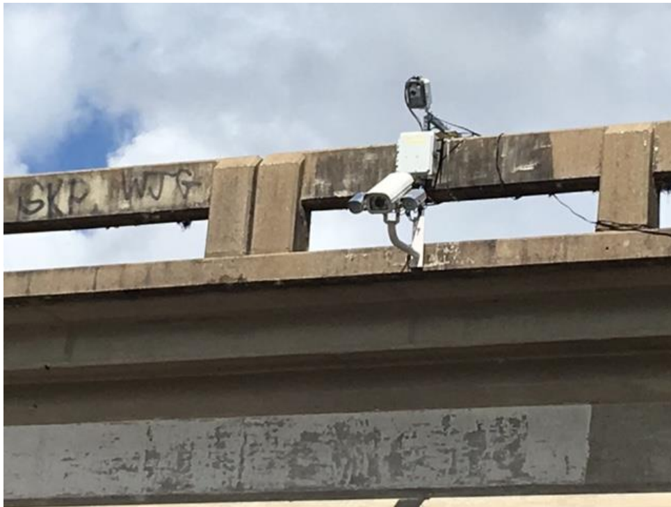
Figure 4-8: Bracket Close-up Showing Sensor, Camera, and Processor
