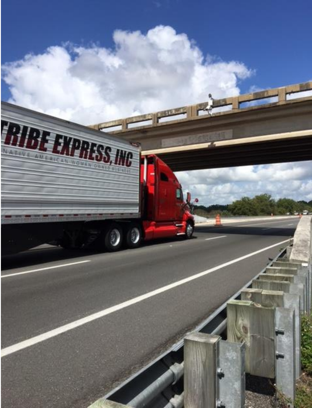
Figure 4-6: Capture System Mounted on Overpass
