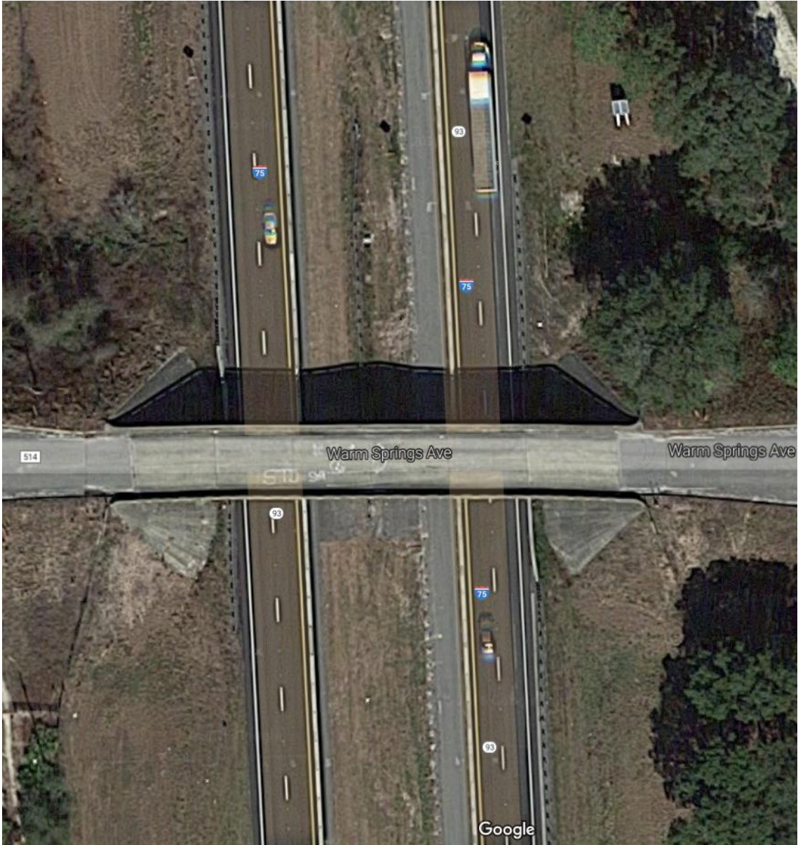
Figure 4-5: Location 3 on I-75 at Warm Springs Ave.
