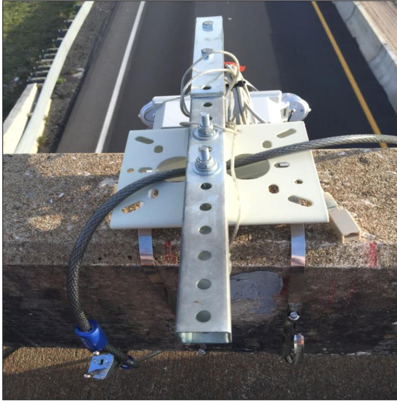
Figure B-0-7: Bracket Connection to Overpass
