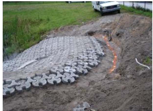
Figure 47: Anchor trench along top of S-139 and S-145
