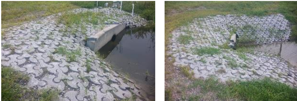
Figure 49: Tri-Lock erosion blocks around S-139 and S-145 80 days following installation
