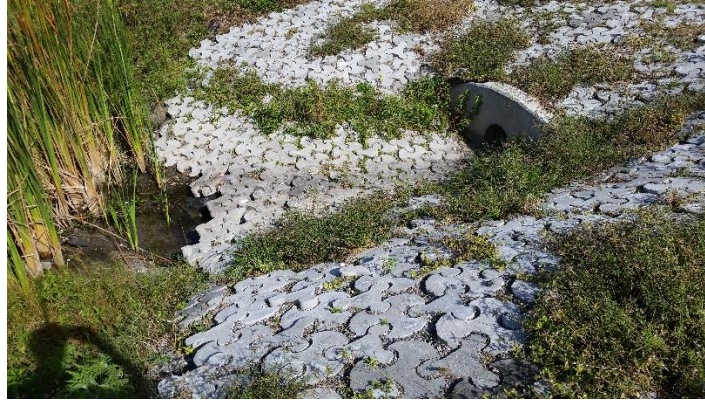
Figure 51: Tri-Lock and vegetation growth around inlet 1
