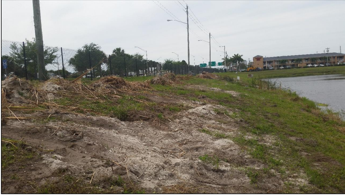
Figure 54: Construction activities at the Royal Palm pond
