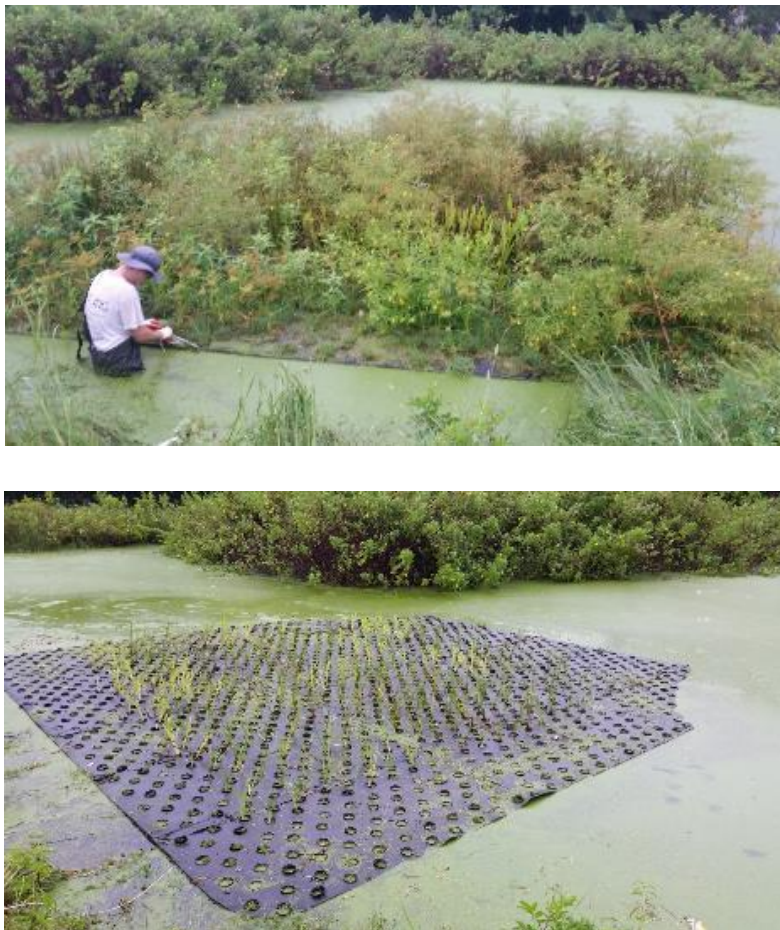
Figure 41: Plant replacement of Ruskin FTW, before (above) and after (below)
