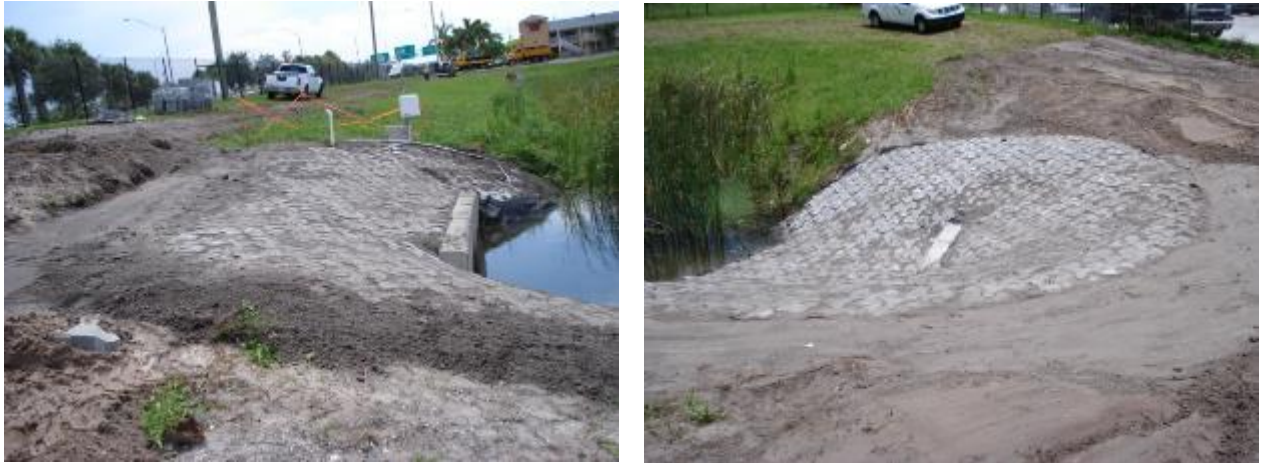
Figure 48: Finished installation of Tri-Lock around S-139 and S-145
