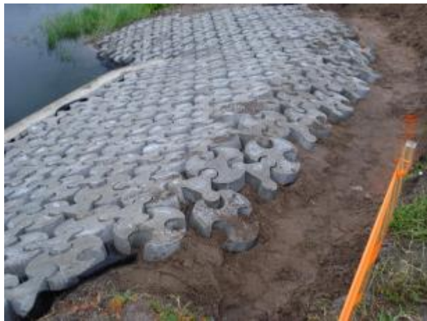
Figure 47: Anchor trench along top of S-139 and S-145
