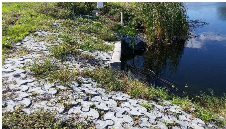
Figure 52: Tri-Lock and vegetation growth around inlet 2
