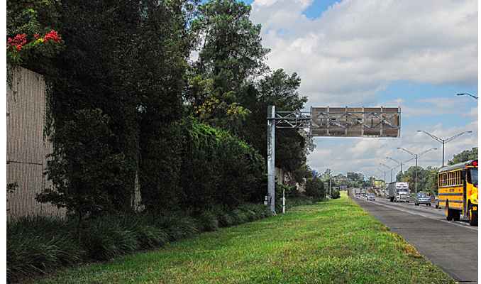
Sound walls, like this one along I-95 in Jacksonville, protect surrounding neighborhoods from the constant road noise of this busy highway.
