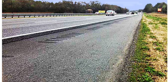
FC-5 asphalt concrete is the widely used on high speed, multilane roads in Florida.
