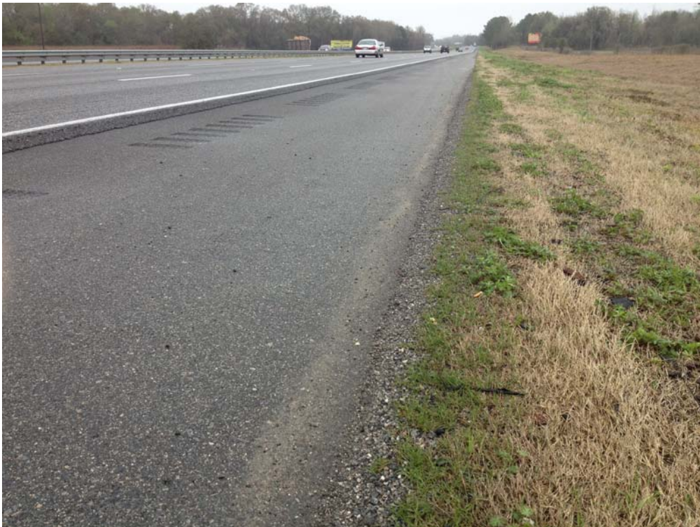
Figure 3.18 - Raveled Aggregates on Shoulder, I-75 Hamilton County (MP 461-462)
