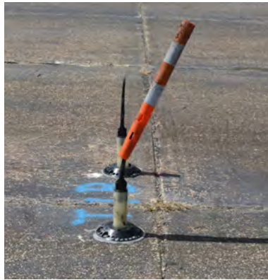
Figure A-1. Sample 1T Failure at 53 Impacts.
