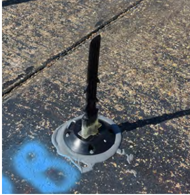
Figure A-14. Sample 7B Failure at 18 Impacts.
