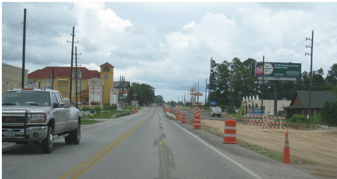
Figure 1-3. Example of an Urban Roadway Work Zone in Texas
