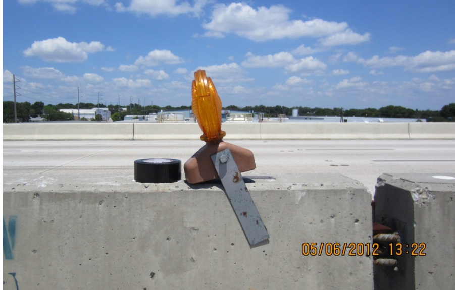
Figure 3-16. Example of Warning Light Misalignment on Temporary Barrier Wall.
