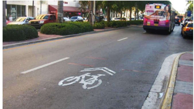
In this pilot study, the bike-and-chevron marking was placed in the center of the outside lane to encourage bicyclists to take over the lane.
