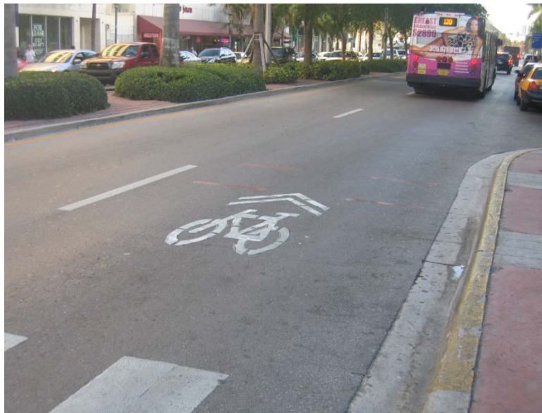
Figure 6. View of sharrow in middle of lane.
