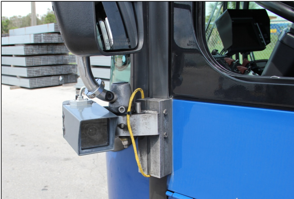
Figure 4-1. Left side camera installed on type A bus.
