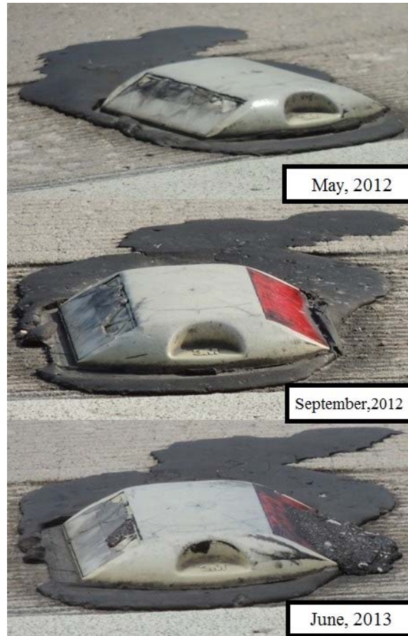
Figure 4-15 3M Marker No.2 at Site 15 (Causeway Blvd & S 50 th St.)
