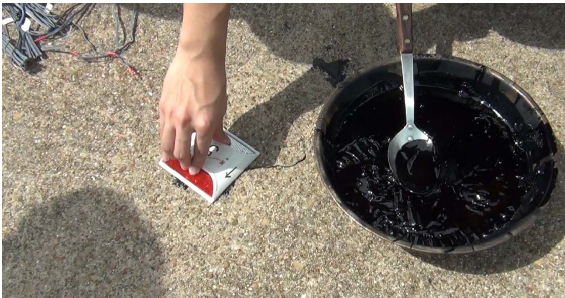
Figure 7-3 Installation of Rayolite RS Marker at the Test Site
