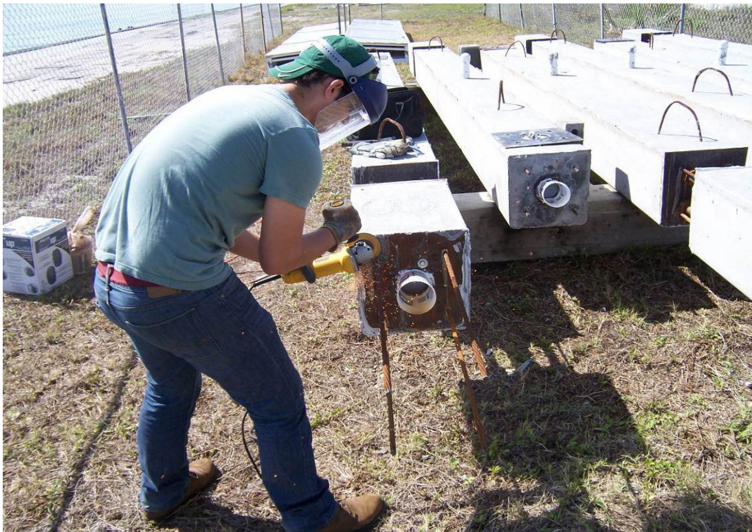
Figure 7 Cutting of Excess Strand Material
