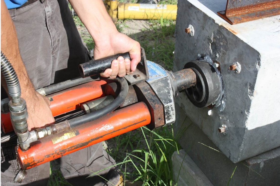
Figure 23 Hydraulic Jack Setup for Stressing Operation Test
