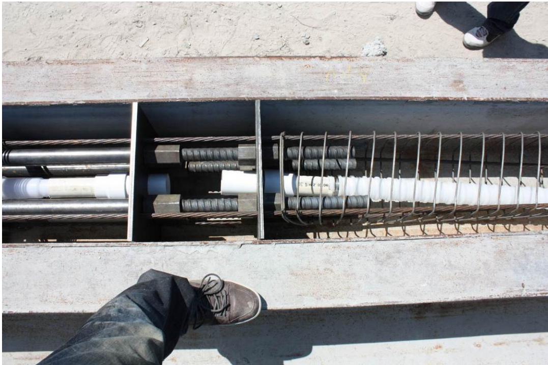
Figure 4 Spiral Wire for Casting of De-Tensioning Piles
