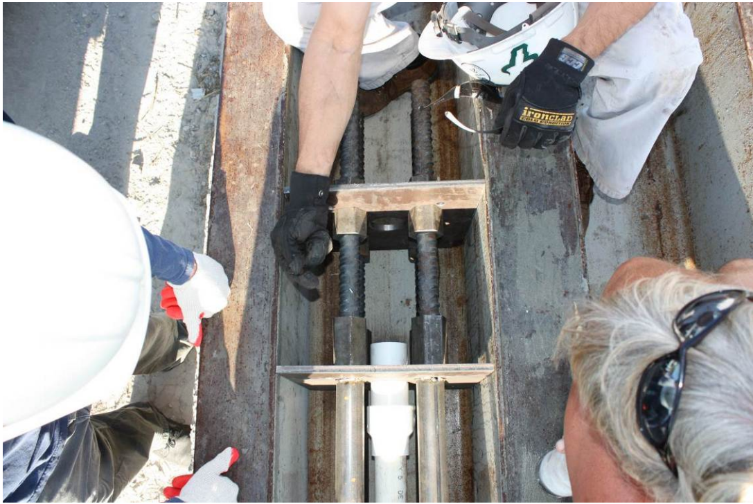
Figure 2 Setup for Casting of De-Tensioning Piles
