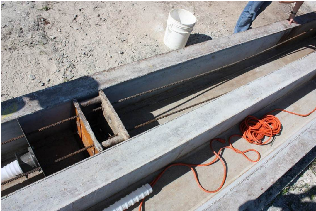
Figure 3 Prestressing Strand for Casting of De-Tensioning Piles
