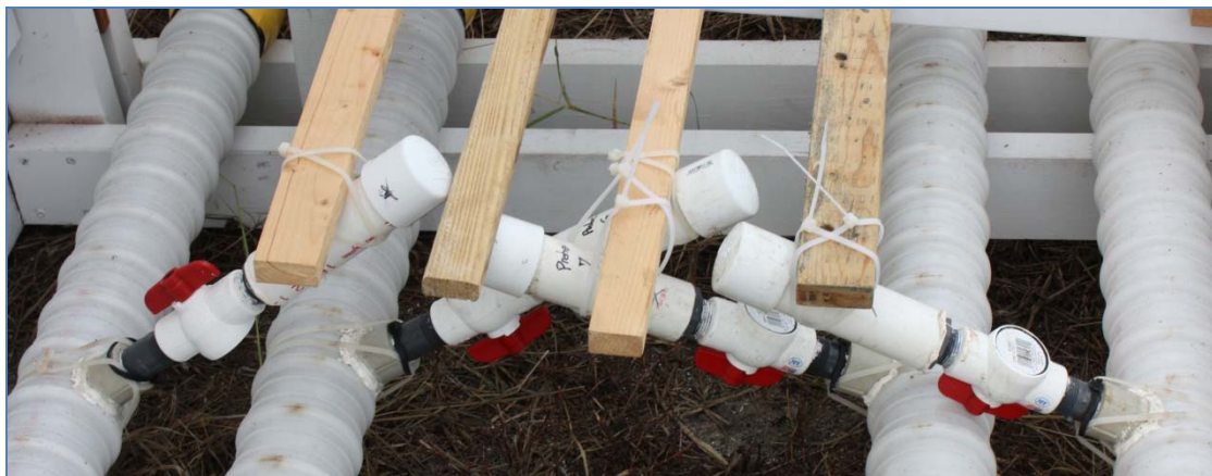
Figure C3 Relative Humidity & Temperature Probe Housings Attached to Ducts via Vent Port and Secured with Wood Boards and Zip-Ties
