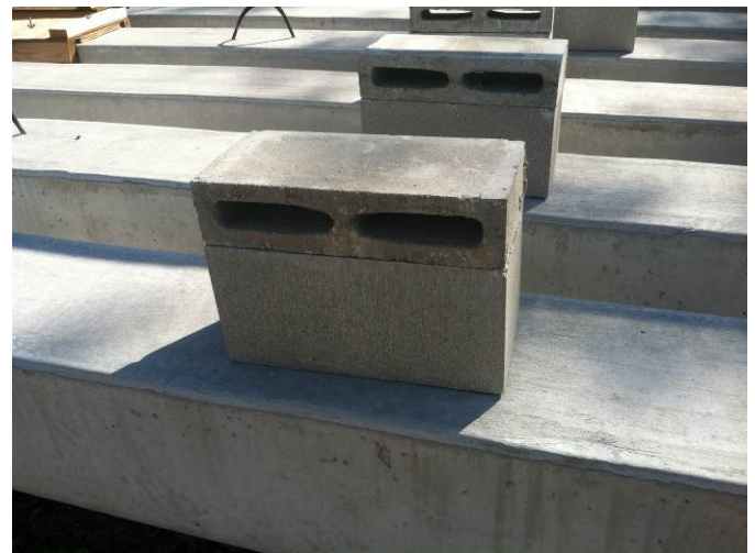
Figure 21 RH Access Port Cinder Block Covers, with Lid
