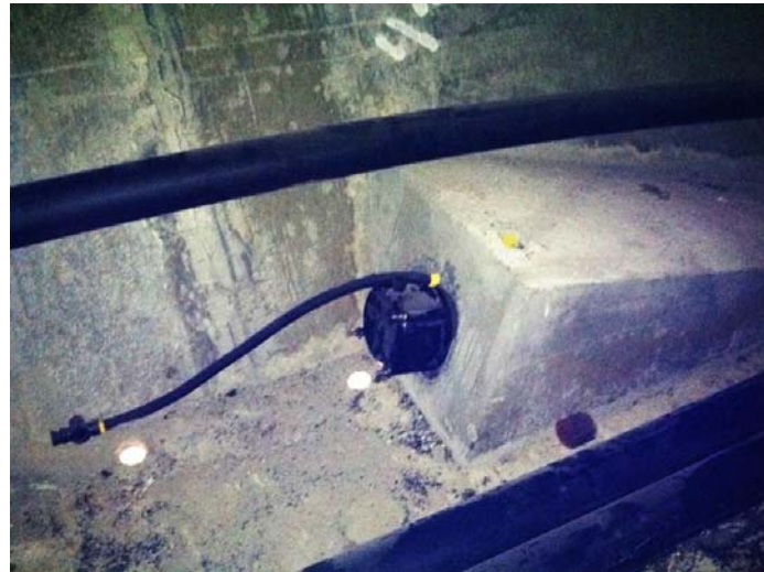
Figure A3 Permanent plastic end cap and grouting port in span 10-8
