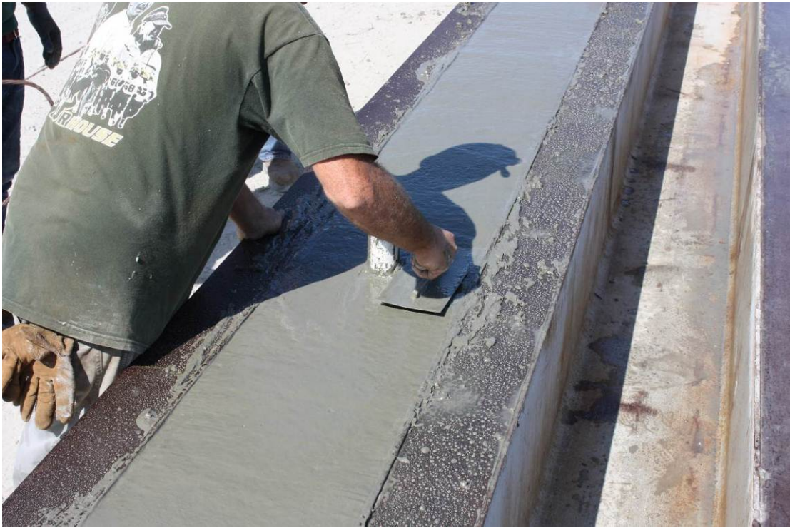
Figure 6 Smoothing of Poured Concrete De-Tensioning Piles
