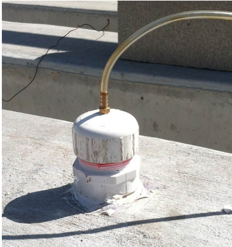
Figure 25 Vacuum Hose Attached to RH Access Port for Vacuum Pressure Testing
