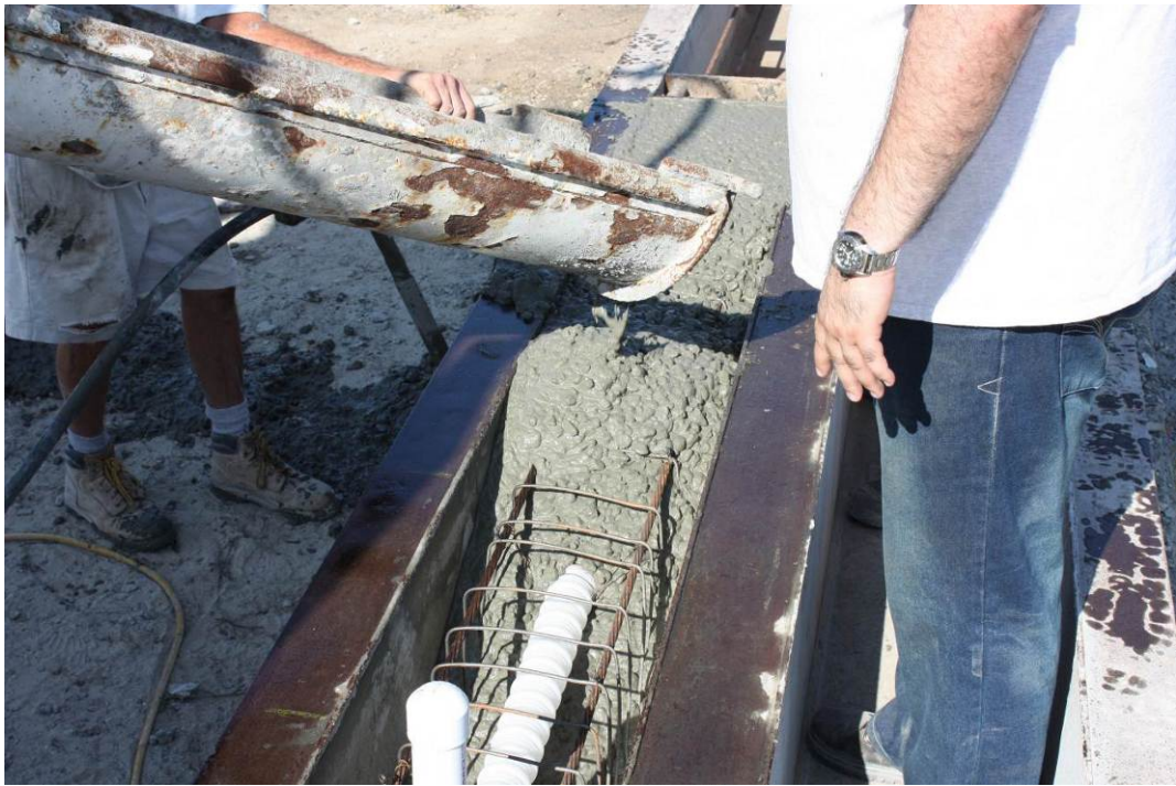
Figure 5 Concrete Pouring for Casting of De-Tensioning Piles
