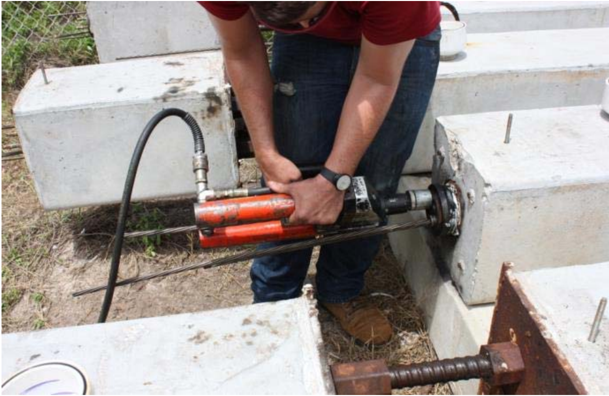
Figure 31 Mono-Strand Jack Used to Stress Strand
