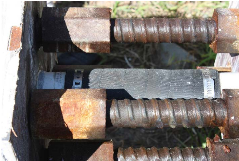
Figure 14 Installed "Bellows" Connection for Pile Segment Break
