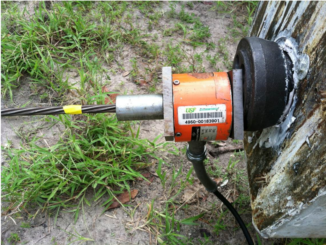
Figure 22 Load Cell Setup for Stressing Operation Test
