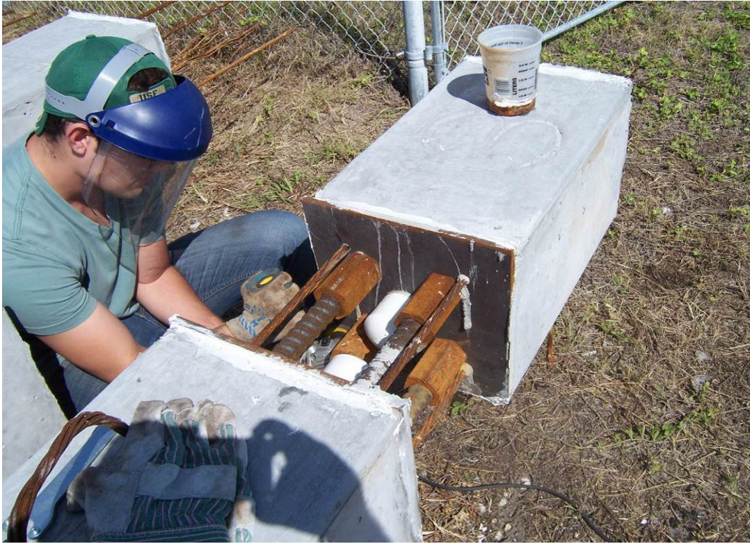
Figure 8 Cutting of Excess Strand Material
