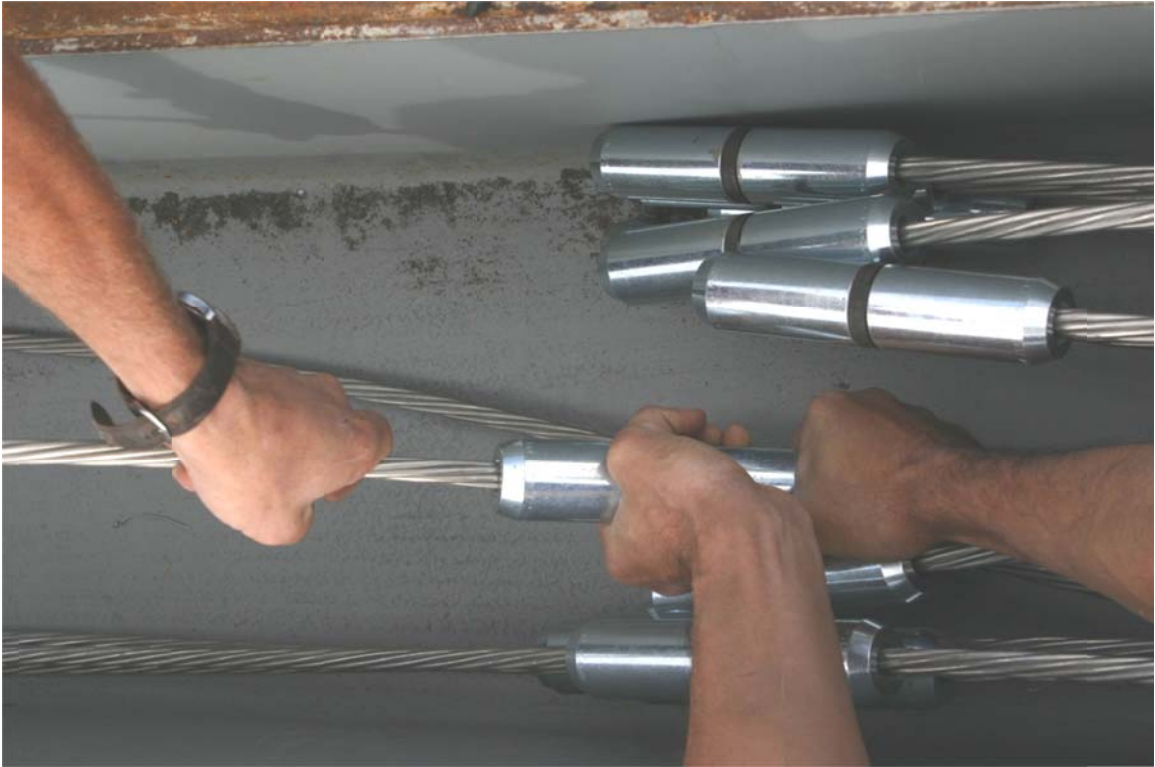
Figure 5.8 Ends of each strand material coupled by splicing chucks.
