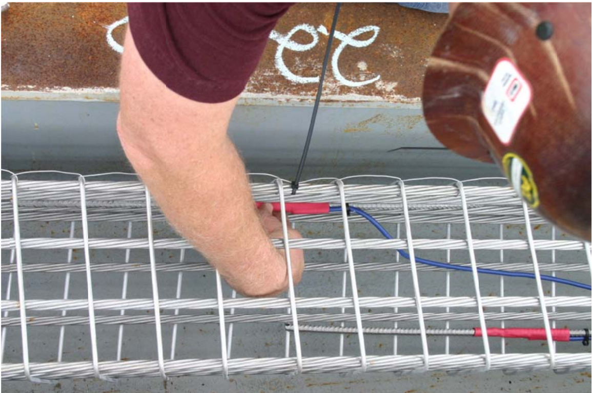
Figure 5.12 Embedded sister bar gages installed at mid height, 28 in from each end.
