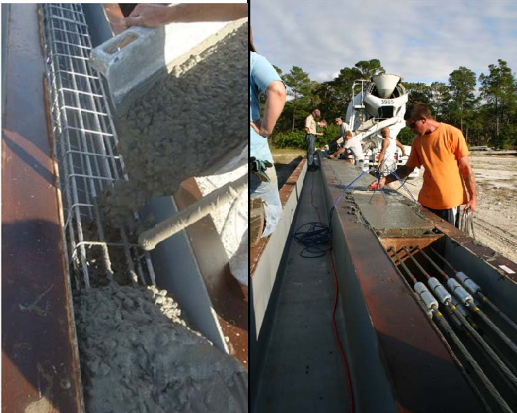
Figure 5.16 Concrete placement and finishing.
