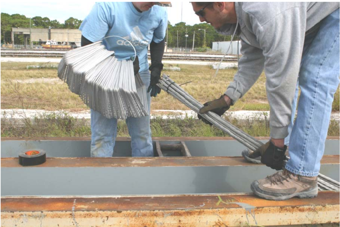
Figure 5.5 Spiral reinforcement placed over cut strands.
