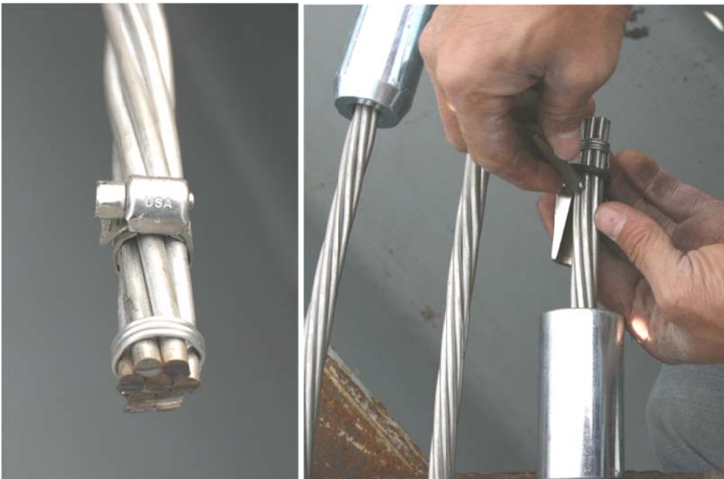
Figure 5.7 Tie wire restrained strand (left); manually inserted in splicing chuck (right).
