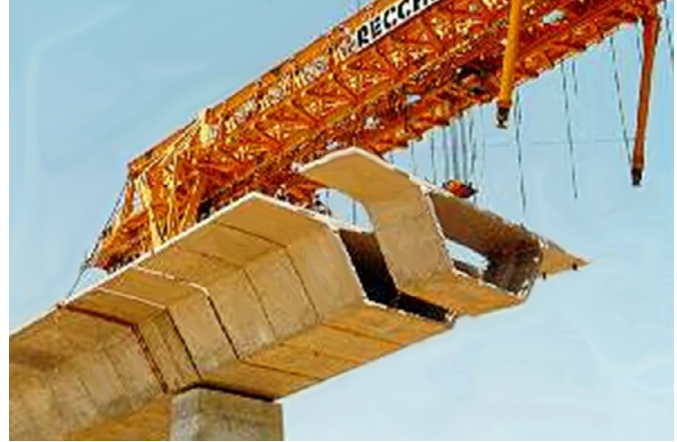
Box girder segments are joined end to end to form bridges. Note the wings that extend to either side of the "box".
