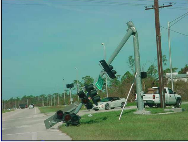
Figure 2.20. Damage to sign structures in Florida during the 2004 hurricane season (Pavlov 2005)
