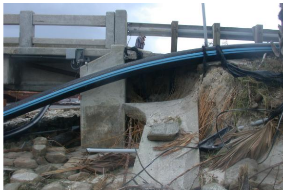
Figure 2.23. Slope failures at bridge bents after Hurricane Jeanne (Danielsen 2012)
