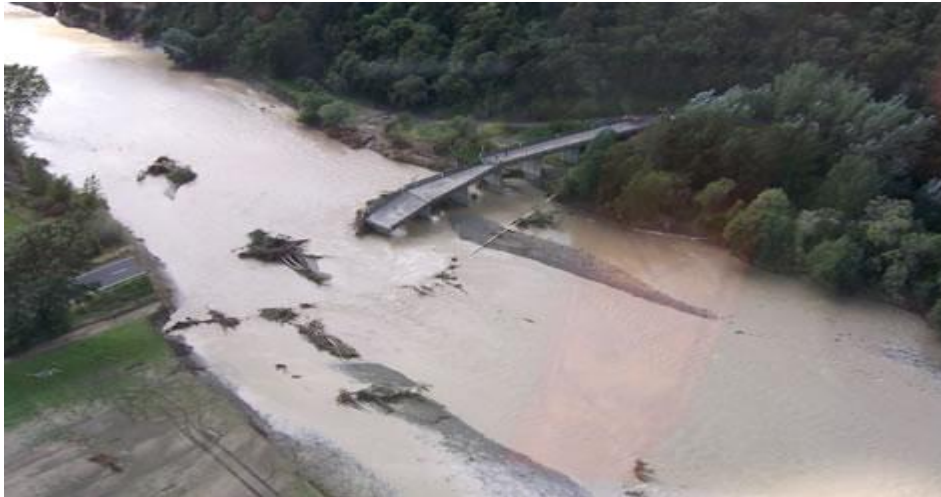
Figure 5.1. The Ashhurst Bridge, Manawatu, New Zealand (Seville and Metcalfe, 2005)
