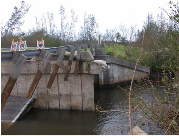
Figure 2.22. Damage to the Mud Creek Bridge after Hurricane Frances (Danielsen 2012)
