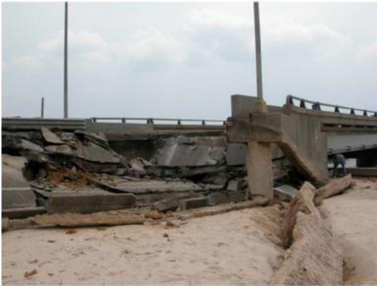
Figure 2.8. Abutment and approach damage from scour and erosion (a) courtesy of MDOT; (b) courtesy of LADOT (Padgett et al., 2008)
