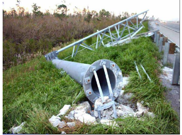
Figure 2.20. Damage to sign structures in Florida during the 2004 hurricane season (Pavlov 2005)
