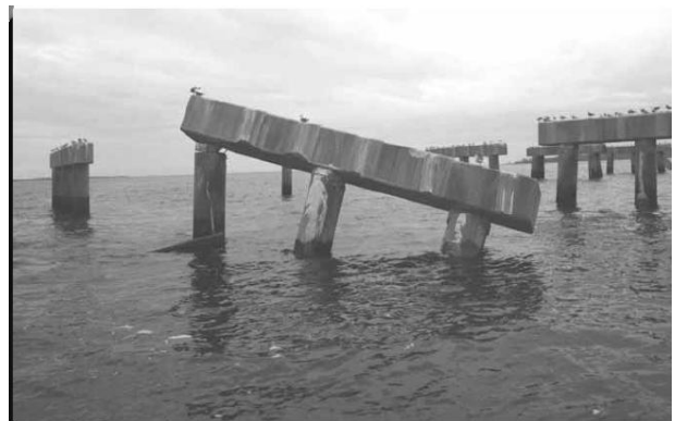
Figure 2.21. Damage to the decks, superstructure, and substructures on I-10 Escambia Bay Bridge after Hurricane Ivan (Maxey 2006)
