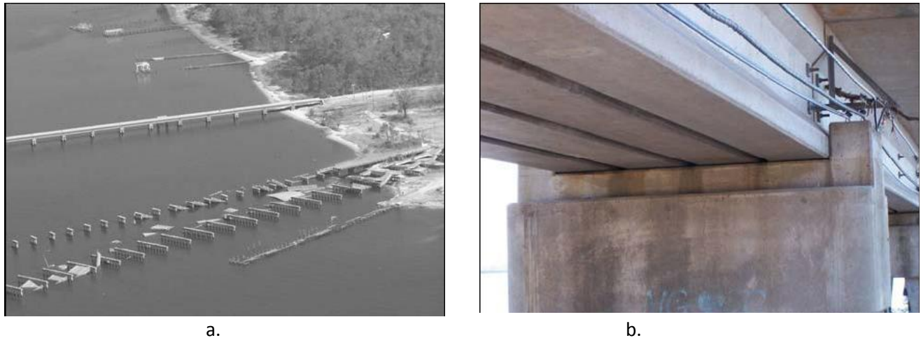
Figure 2.24. Bridges over Biloxi Bay: (a) two bridges severely damaged but parallel railroad bridge remained standing (b) lateral restraints (Gilberto et al., 2007).
