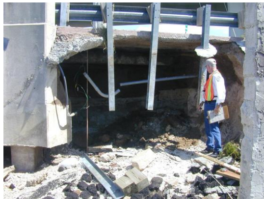
Figure 2.23. Slope failures at bridge bents after Hurricane Jeanne (Danielsen 2012)
