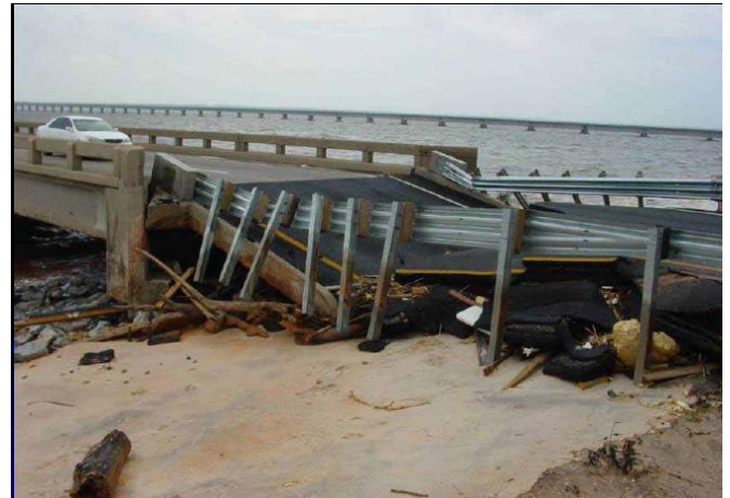
Figure 2.19. Damage to bridge approach slabs in Florida during 2004 hurricane season (Pavlov 2005)
