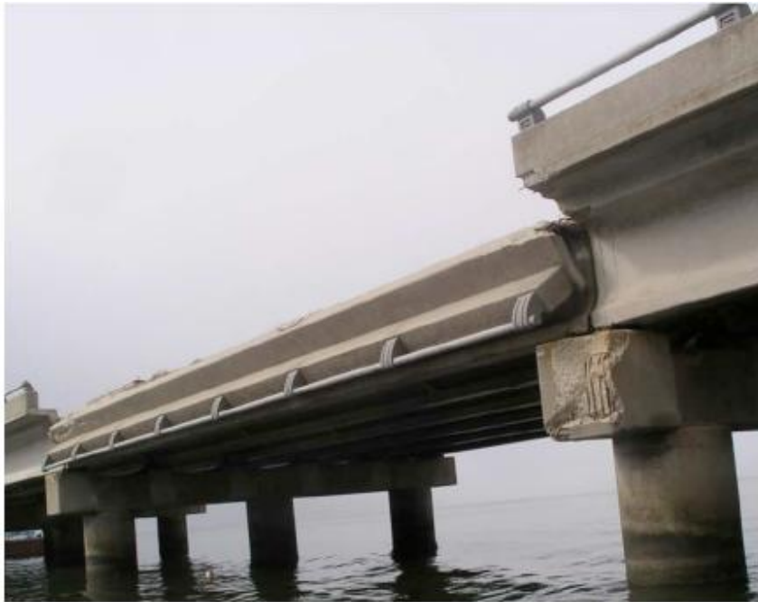
Figure. 2.6. Damage to bent caps (a); bridge parapet (b) due to storm surge (Padgett et al., 2008)
