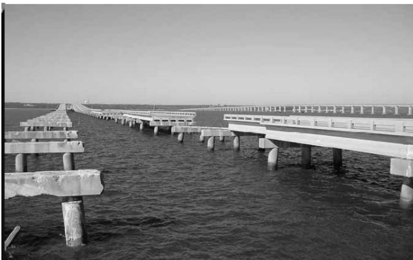
Figure 2.21. Damage to the decks, superstructure, and substructures on I-10 Escambia Bay Bridge after Hurricane Ivan (Maxey 2006)
