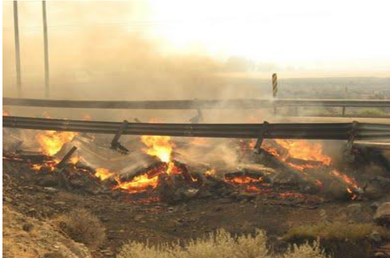
Figure 7.21. Fire consumption of timber bridge Washington State – WSDOT
