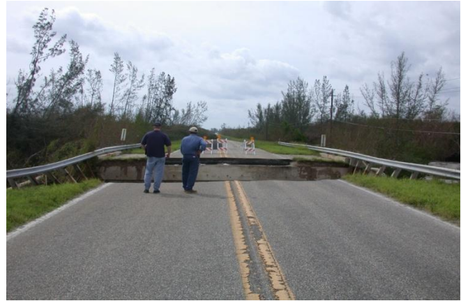
Figure 2.22. Damage to the Mud Creek Bridge after Hurricane Frances (Danielsen 2012)
