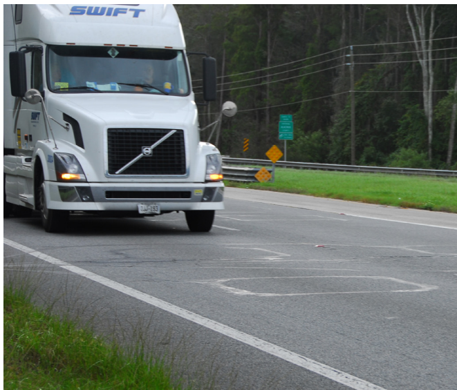
A semi is about to drive over an electromagnetic loop embedded in the pavement. The loop is one component of a traffic monitoring site.
