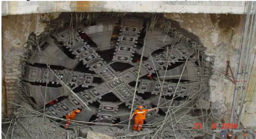
Figure 2.11: TBM cutting through FRP-reinforced concrete drilled shaft wall
