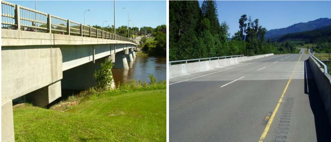
(a) Joffre Bridge (b) Waterloo Creek Bridge Figure 2.5: Pictures from the five field demonstration projects considered
