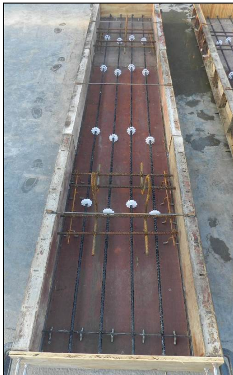
Figure 5.215: Assembled concrete form with BFRP bars and steel lifting hooks
