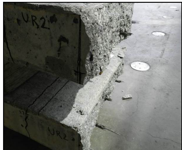
Figure 5.223: Total collapse of the under-reinforced slab and failure of the BFRP reinforcement
