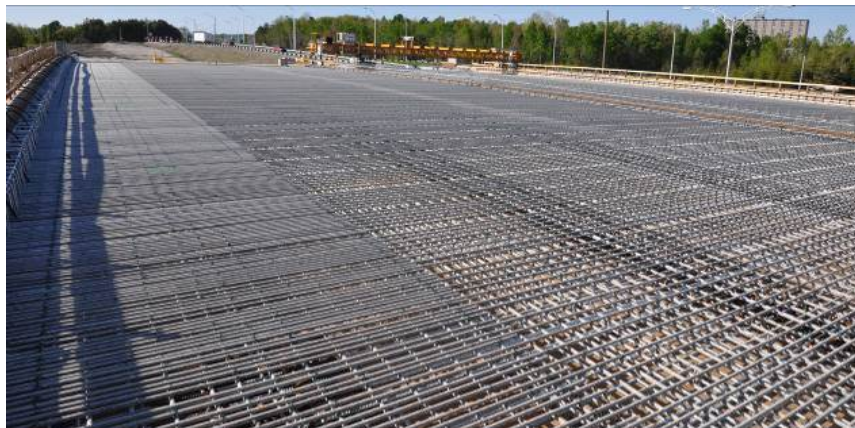
(c) Reinforcement of the bridge deck, 410 overpass bridge Quebec, Canada Figure 2.9: Recent FRP-reinforced concrete bridges
