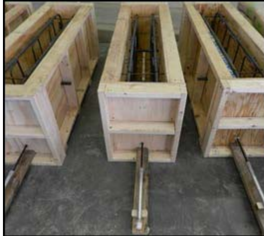
Figure 5.194: Completed formwork
