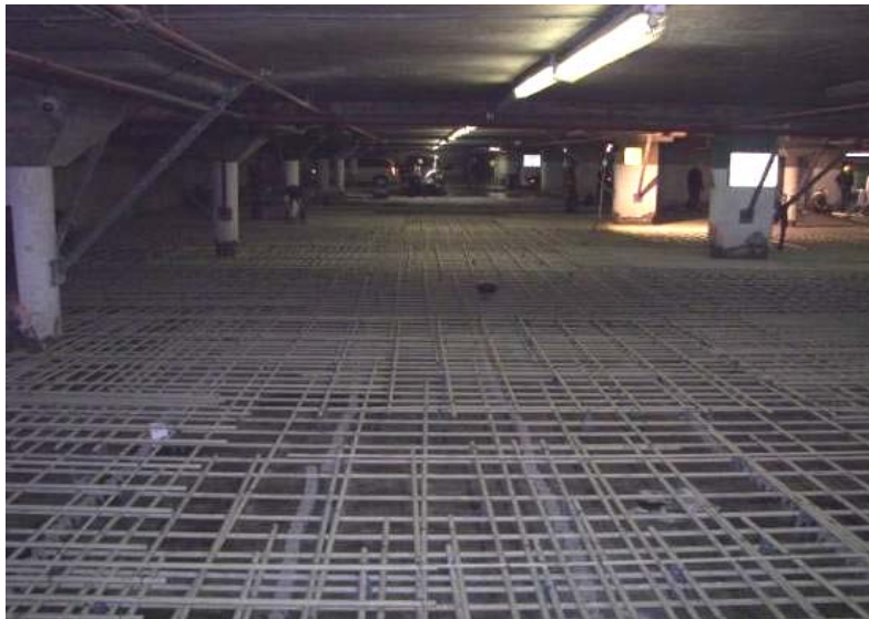
Figure 2.14: La Chancelière Parking Garage
