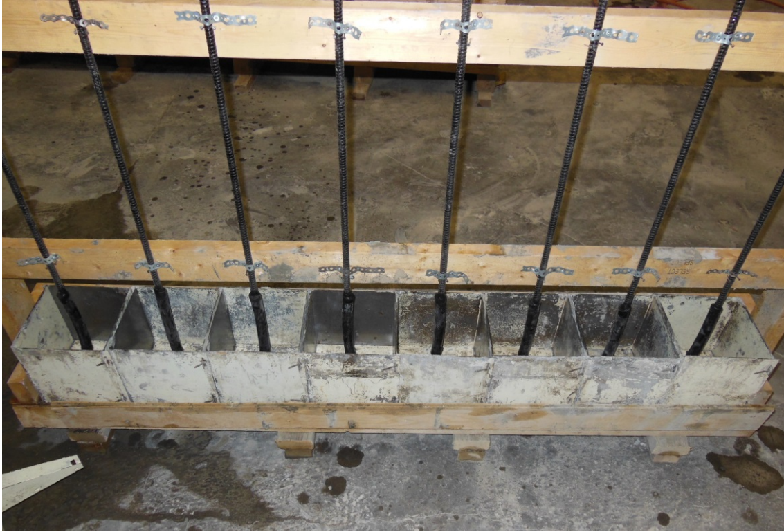
Figure 5.24: BFRP bars inside the block formwork
