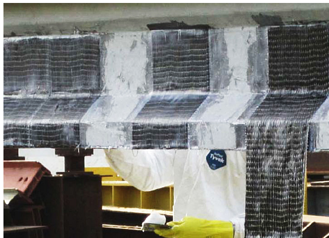
A technician works on wet layup application of CFRP fabric laminate on a prestressed concrete girder.
