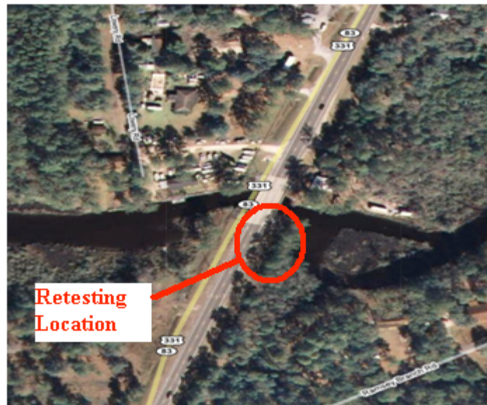
Figure 2.13 Aerial View of Ramsey Branch Bridge at Freeport, Florida (from Google Maps)
