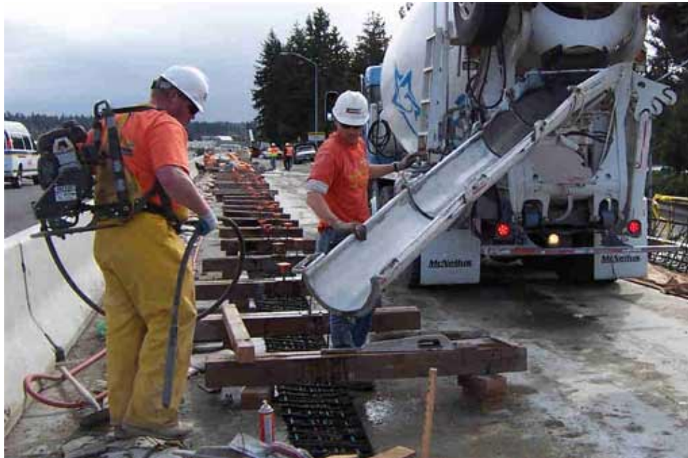
Figure 1-1. Casting the closure region between phases.
