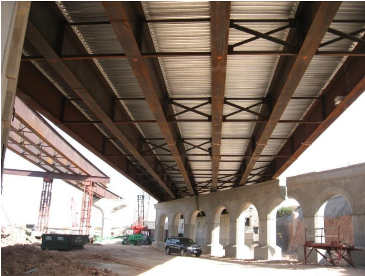
Figure 4.11: Lean-on bracing system in 19 th Street Bridge
