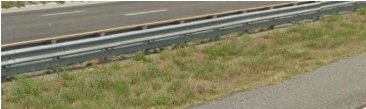
Figure 1-2: G4 (1S) Strong-post W-beam Guardrail with a Rub-rail on I-95 in St. Johns County
