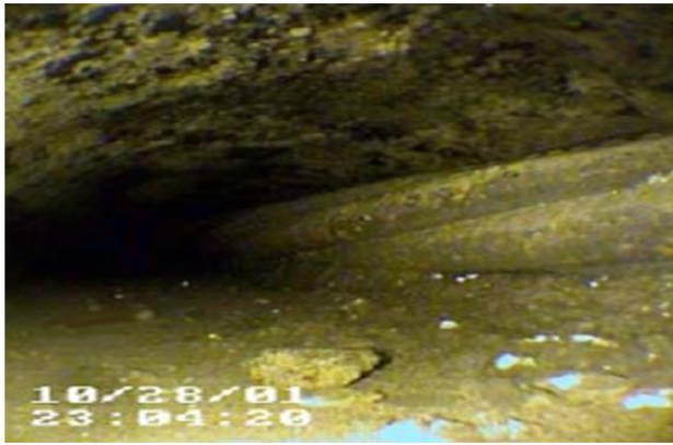
Partially grouted duct
