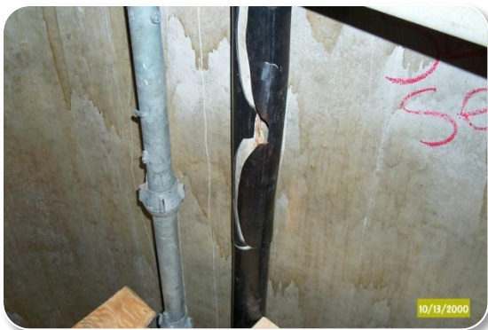
Figure 1.6: Examples of types of observed cracking of ducts
