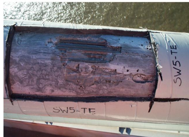
Figure A.2: Examples of hands-on inspection of cable with a traveling buggy (left) and a dissected cable, revealing exposed steel cable wires (right)
