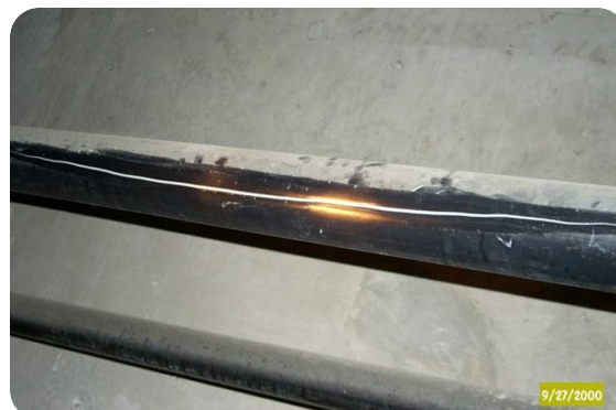
Figure 1.6: Examples of types of observed cracking of ducts
