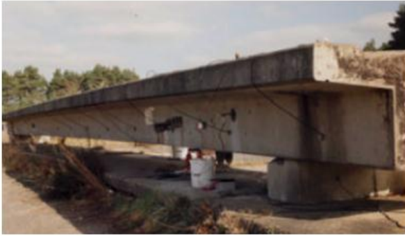
Instrumented Bank Lane Unit
