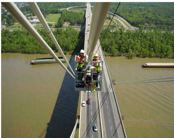
Figure A.2: Examples of hands-on inspection of cable with a traveling buggy (left) and a dissected cable, revealing exposed steel cable wires (right)
