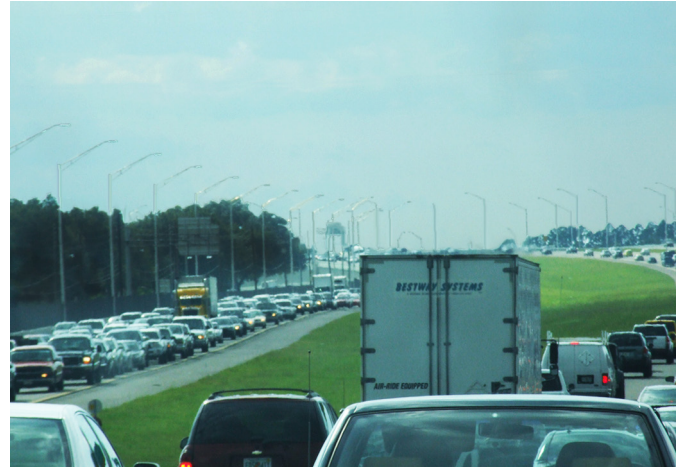
A typical day on I-4 in Orlando. The interstate corridors in Florida are often congested, costing users time and money.
