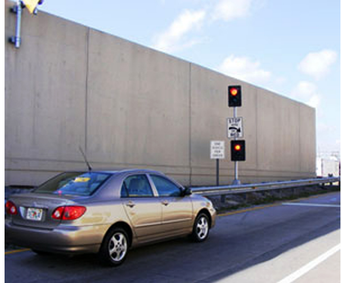
A car waits at a ramp signal before entering I-95 in South Florida. Regulating the rate at which cars enter the interstate can improve overall traffic flow on the highway.
