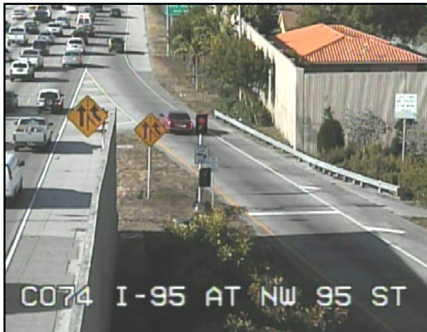
Figure 1-1 A Ramp Signal Implemented by FDOT
