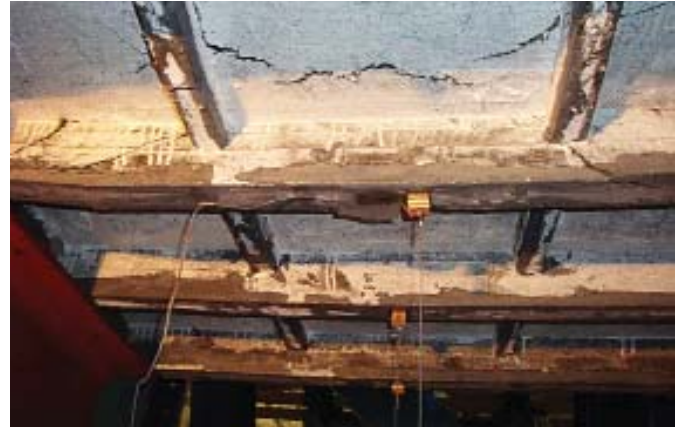
This post-test view of the underside of a UHPC-HSS bridge deck unit in an experimental setup shows the basic deck structure with primary and secondary ribs.
