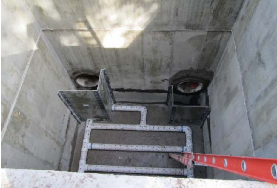
Figure 6-5 Up-flow Off-Line Sorption Filter before Media Placement
