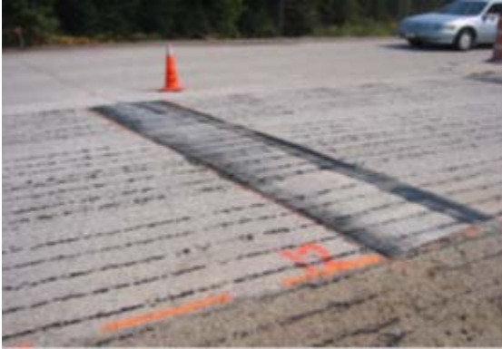
(i) Close-up of the tack coat application
