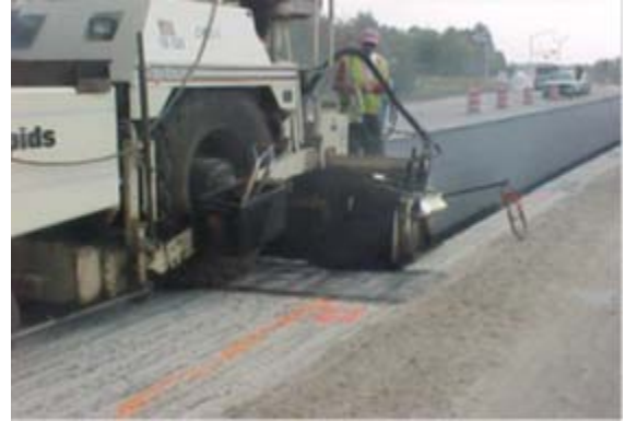
(k) Paving over the ISAC
