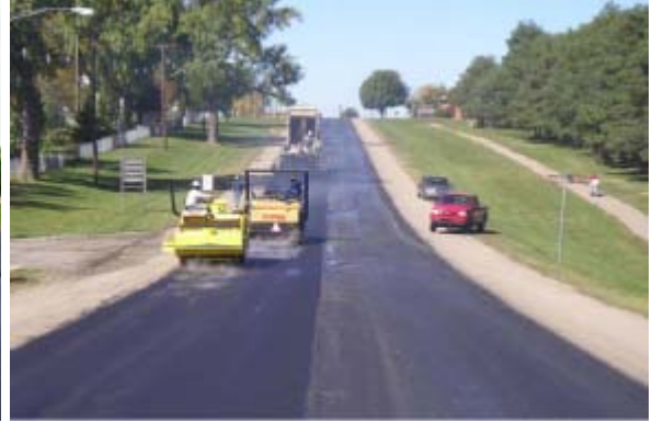
(b) Construction compaction of Strata project (Final stage)
