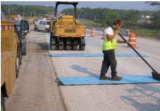
(g) Rolling ISAC pieces with a rubber tire roller
