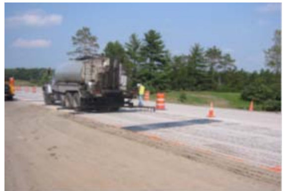
(h) Application of the tack coat prior to paving
