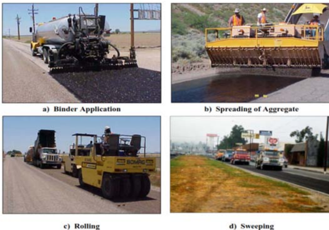
Figure C.5: Construction procedure of chip seal
