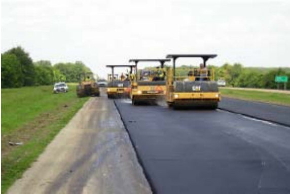
(a) Construction compaction of Strata project (Initial stage)
