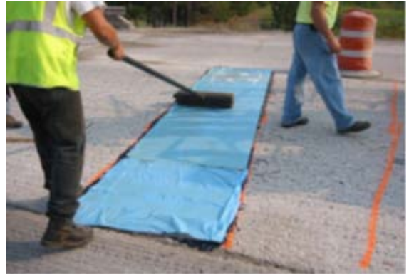
(f) ISAC being rolled with a hand roller
