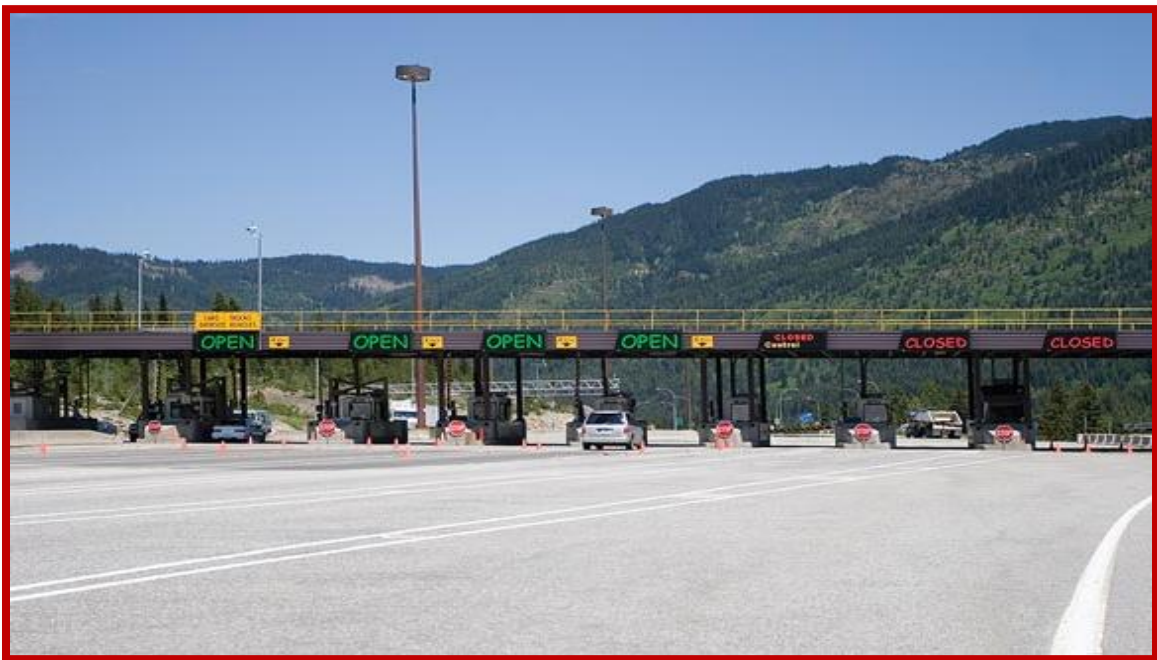
Figure 4-10: Traditional Mainline Toll Plaza (TMTP) (Source: FHWA, 2013)
