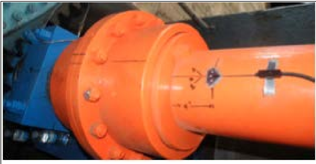
Figure 15-Strain rosette on the drive shaft
