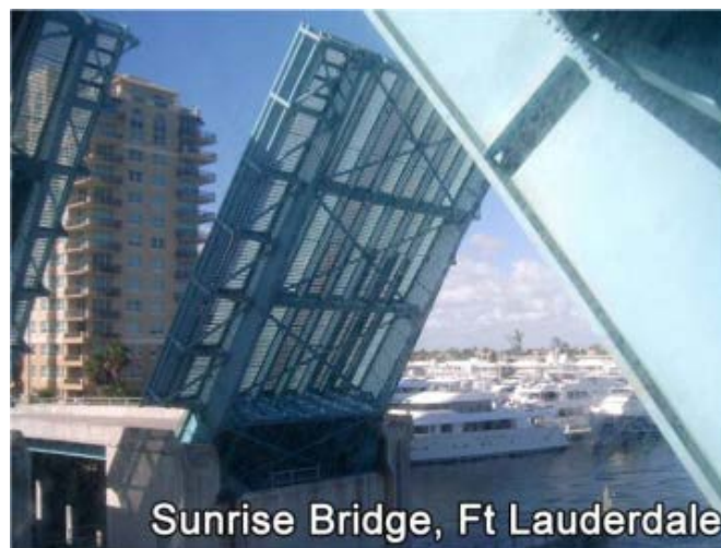
Figure 22-Structural components of Sunrise Boulevard Bridge
