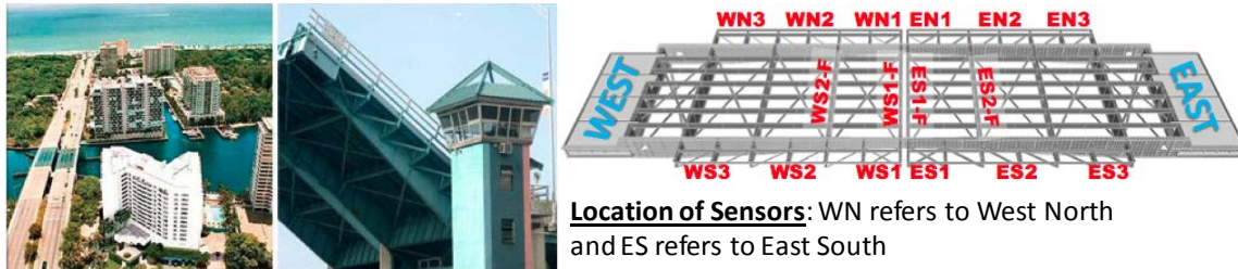
Figure 30-Sensor locations for structural components of Sunrise Boulevard Bridge
