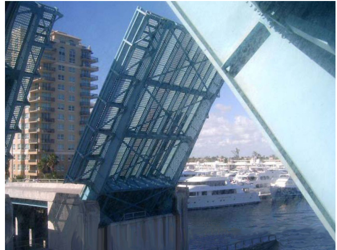
Sunrise Boulevard Bridge in Ft. Lauderdale, shown with its movable leaves in raised position.
