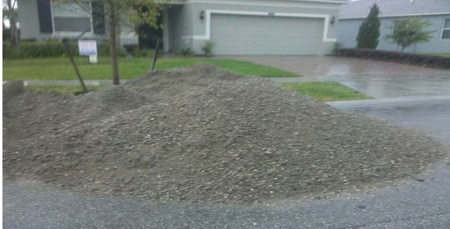
Figure 5: Improper aggregate storage
