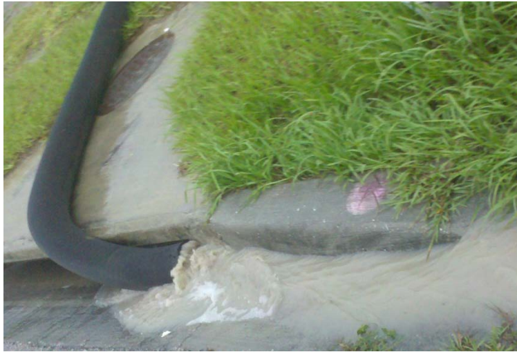
Figure 4: Improper curb inlet protection practice
