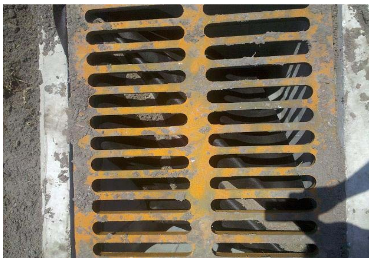
Figure 3: Improper drop inlet protection
