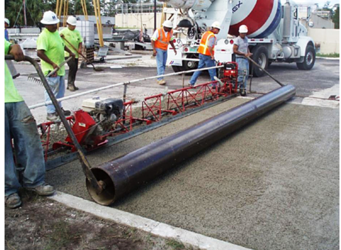
The porosity of pervious concrete paving is achieved through specific installation methods. Here, workers finish the concrete surface with a compactor.
