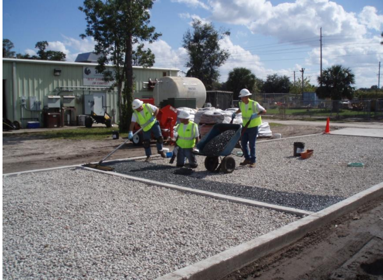
Figure 8: Surface layer installation
