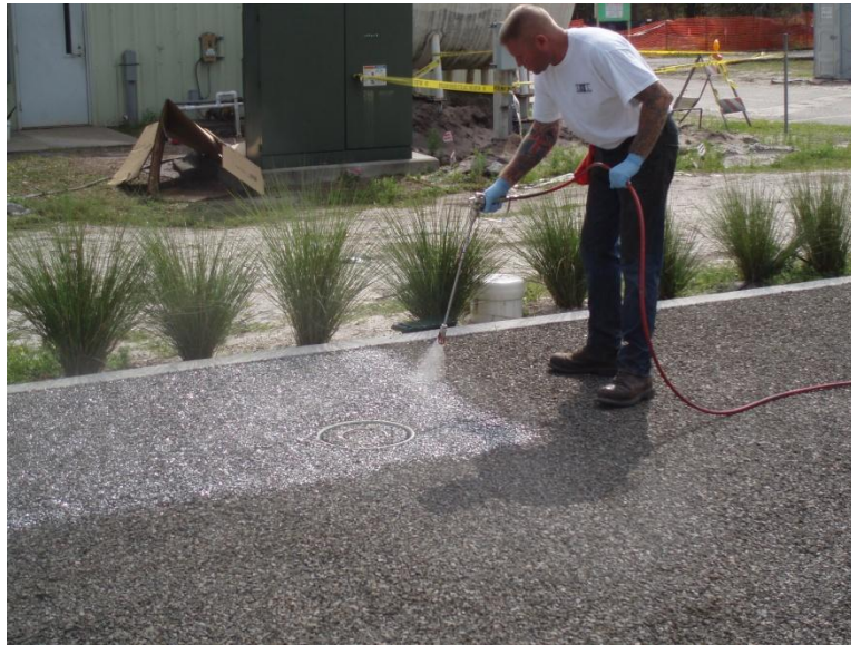
Figure 10: Overcoat application
