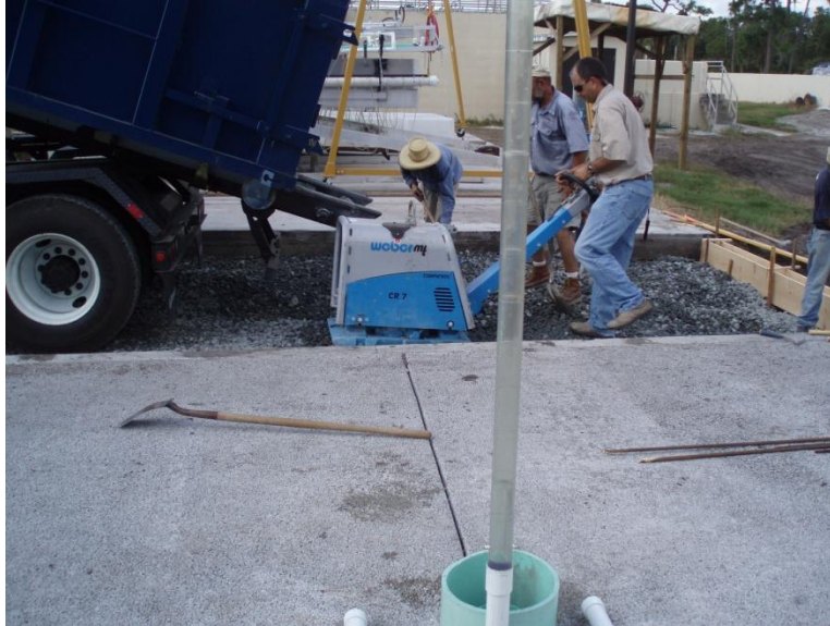
Figure 6: Aggregates placed, leveled, then compacted
