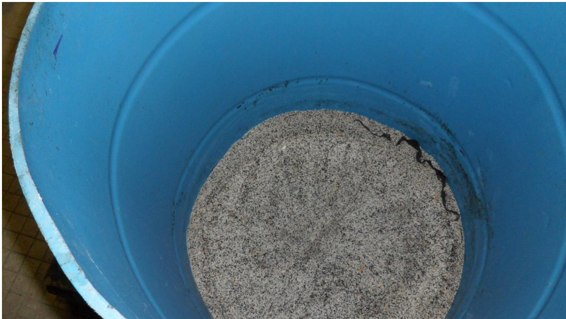
Figure 22: 4 Inches of Bold&Gold™ Pollution Control Media Installed
