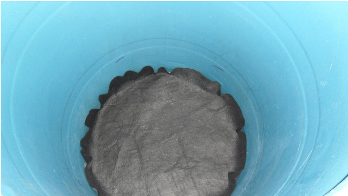
Figure 21: Non-woven Geotextile Separation Fabric Installed
