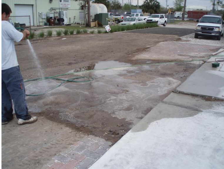
Figure 9: Washing in A-2-4 soils with garden hose
