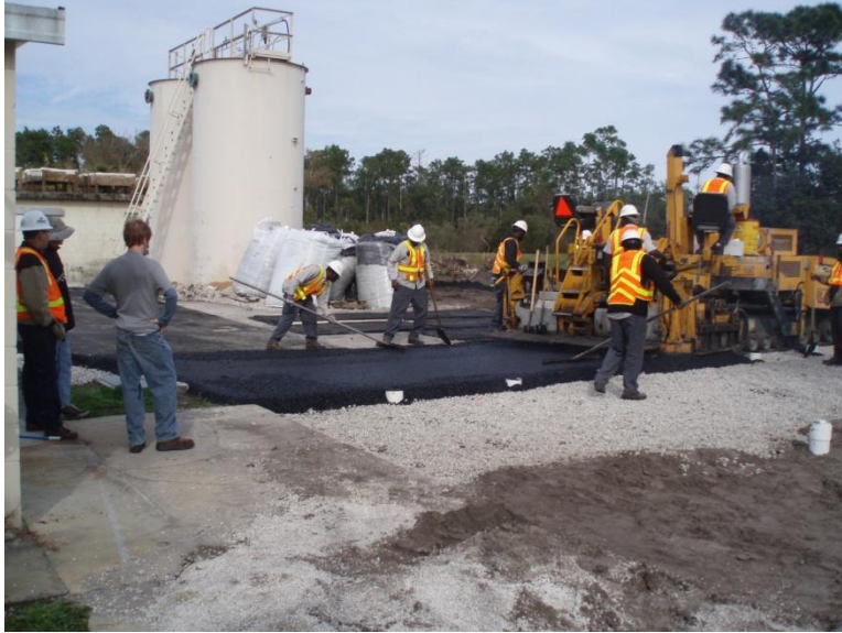
Figure 5: Installation of Pavement layer
