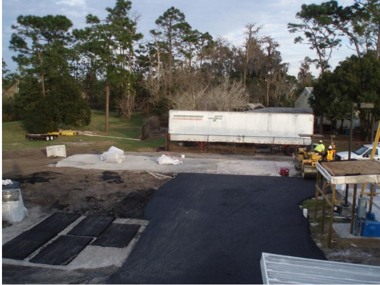
Figure 7: Final layout pavement sections
