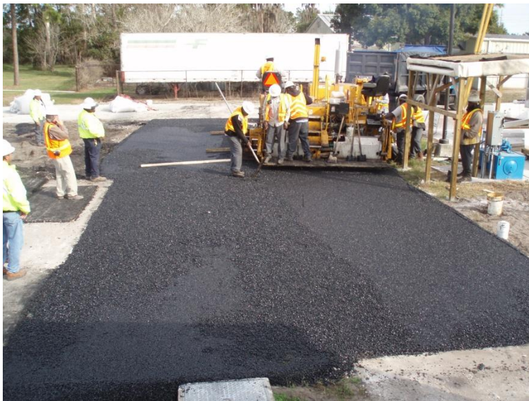
Figure 5: Installation of Pavement layer
