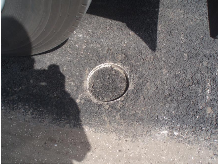
Figure 17: Porous asphalt surface after vacuuming
