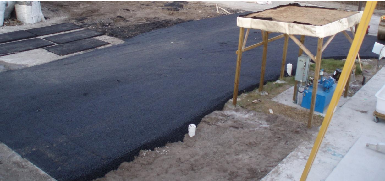
Figure 8: Final Layout of Pervious Pavement Sections with ERIKs
