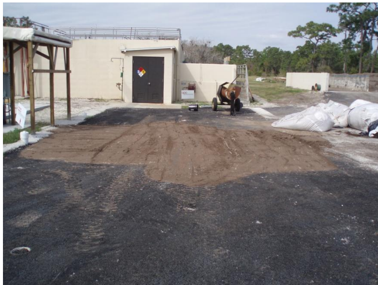
Figure 9: The A-3 sediments spread evenly over entire Rejuvenation section
