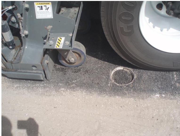
Figure 16: Porous asphalt surface after vacuuming
