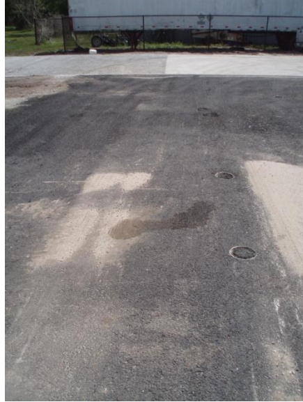
Figure 15: Porous asphalt surface after vacuuming
