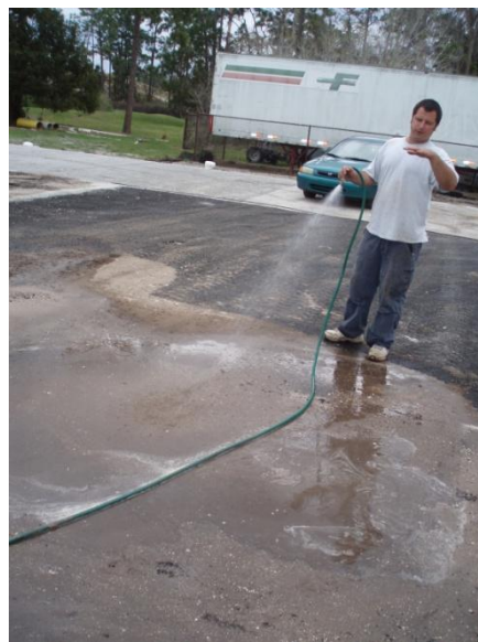
Figure 11: Washing in sediments using garden hose
