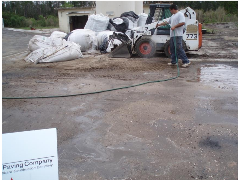
Figure 10: Washing in A-3 soils with garden hose
