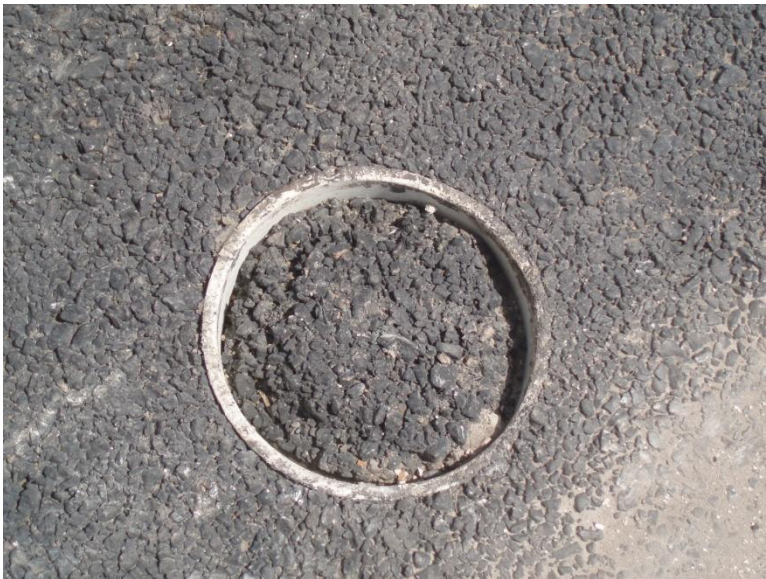
Figure 18: Close up of Porous asphalt surface after vacuuming
