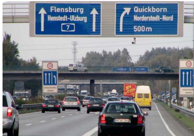
FIGURE 7.4 Termination of Hard Shoulder Use at an Interchange in Germany (source: Kuhn, 2010)
