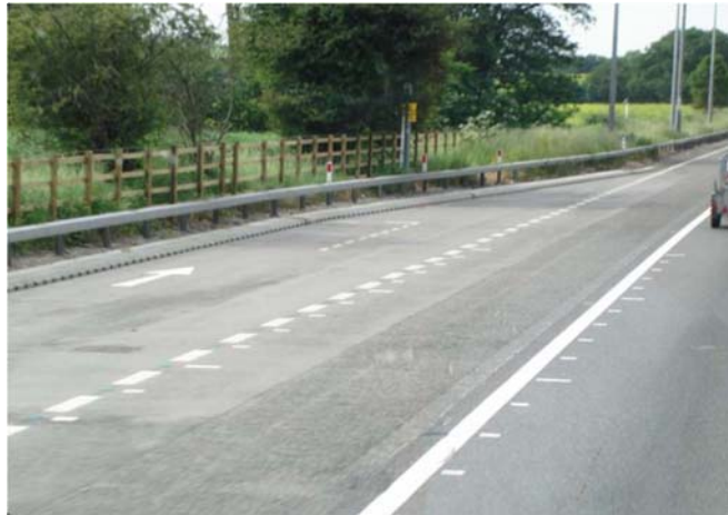
FIGURE 7.7 Emergency Refuge Area on Facility with ATM (source: Kuhn, 2010)
