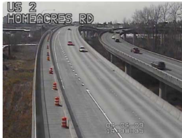
FIGURE 7.11 Shoulder Lane Use on US 2 Trestle in Washington State (source: FHWA, 2010)
