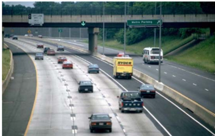
FIGURE 7.8 I-66 Shoulder Lane Use during Peak Periods
