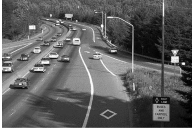
FIGURE 7.12 SR 520 BOS On-Ramp Diamond Weave Markings in Washington State (source: Martin, 2006)
