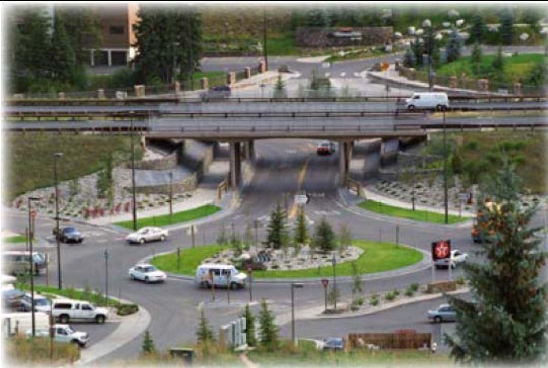
Figure 24. Roundabout at an Interchange (FHWA, 2006, p. 8)
