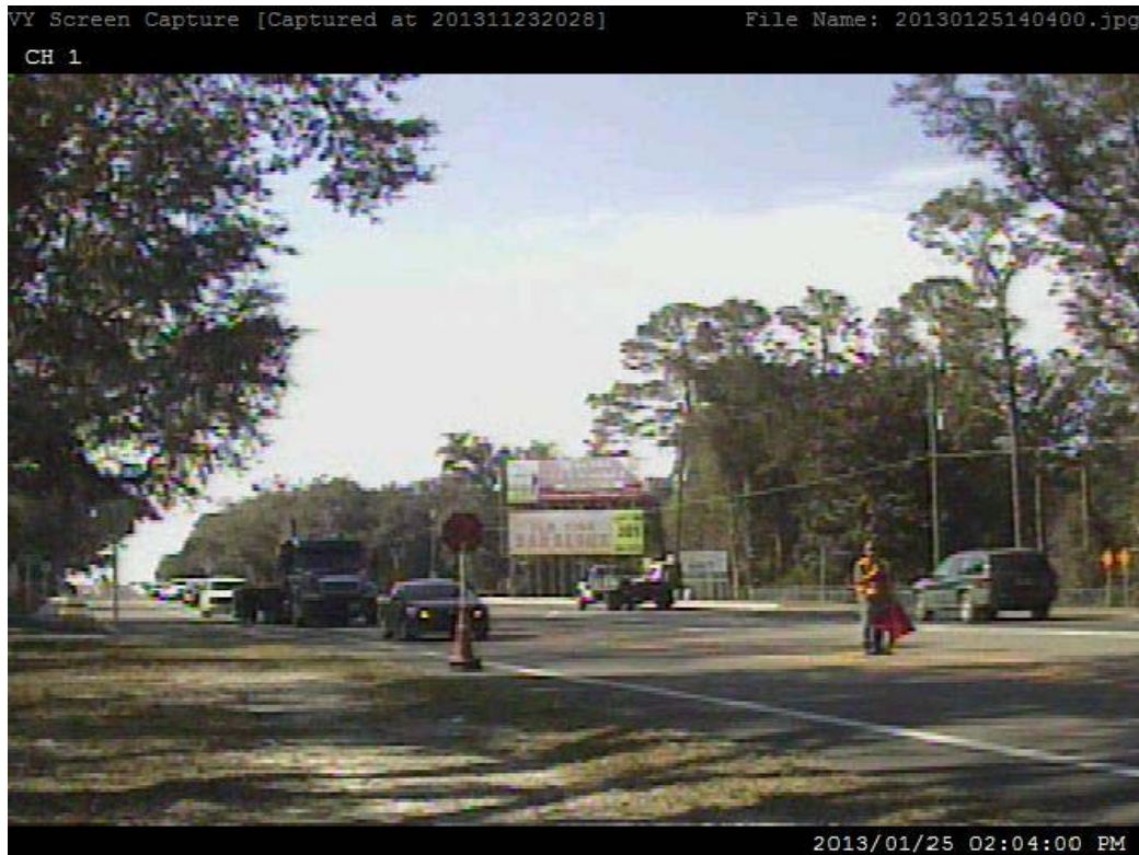
Figure 14. Entrance to work zone at site 3 on 1/25/2013
