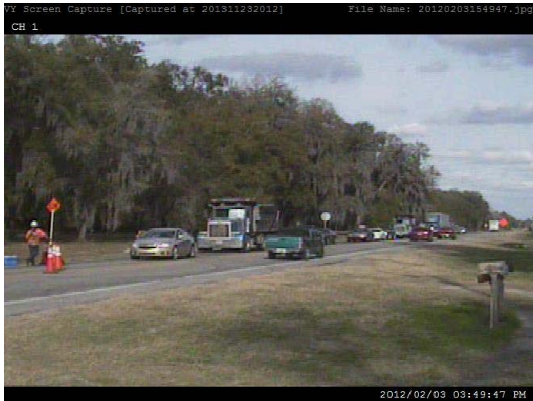
Figure 13. Entrance to work zone at site 2 on 2/3/2012
