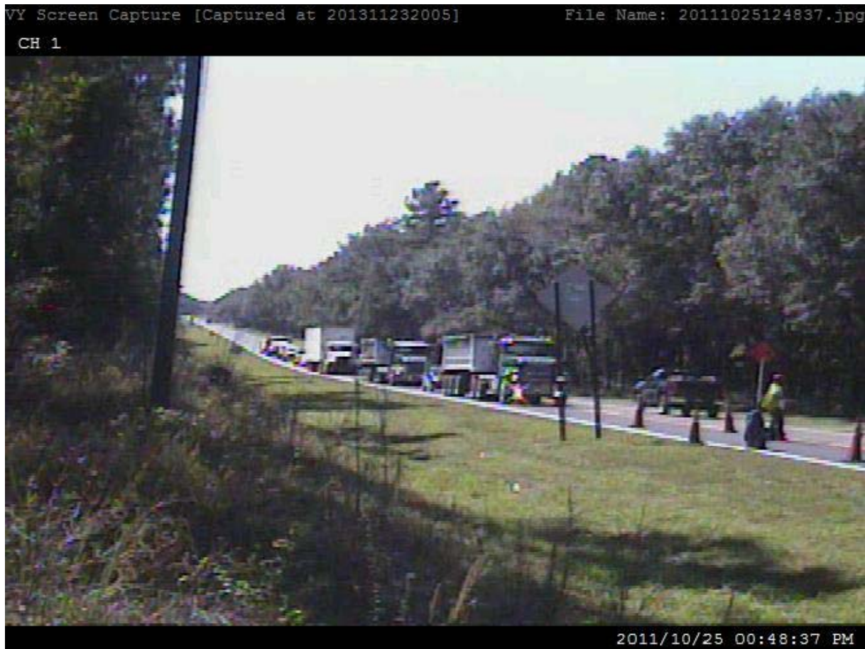
Figure 12. Entrance to work zone at site 1 on 10/25/2011
